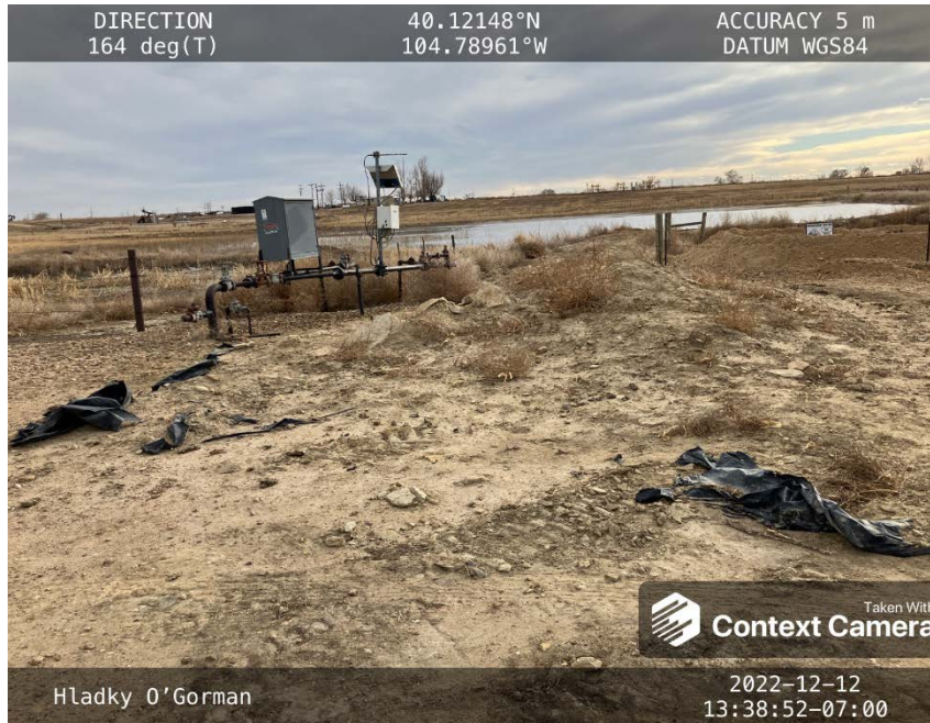
Photo 3 – Liner is beginning to rip under the contaminated stockpile
