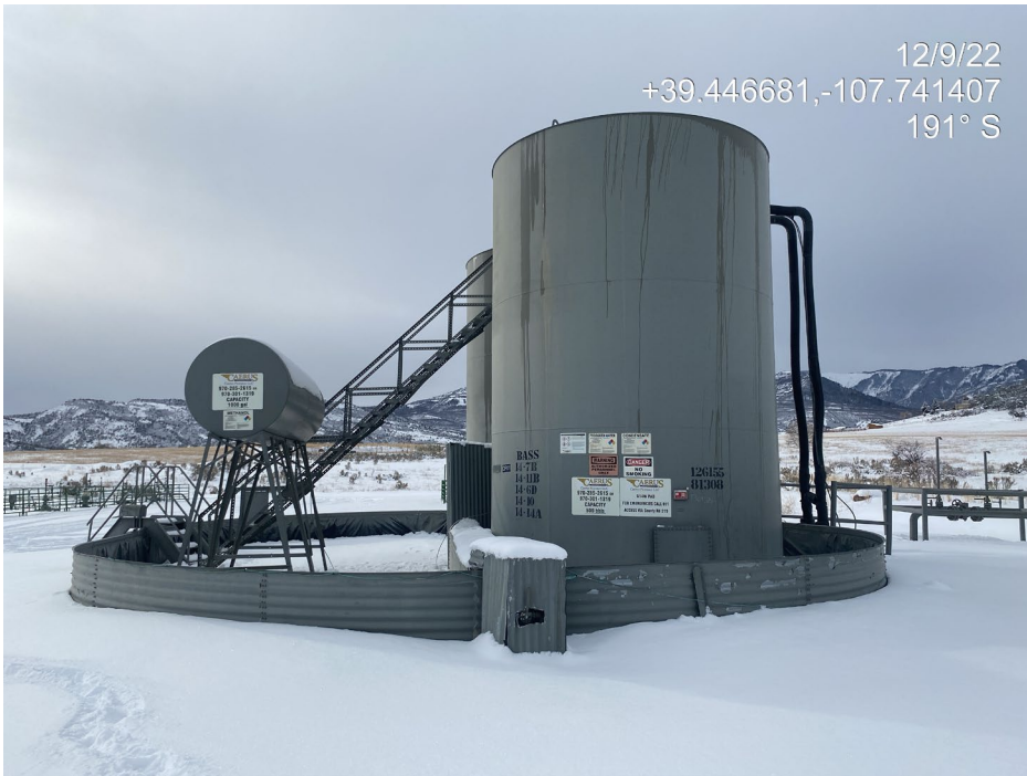
Photo 3. Photos show production areas. Note lack of tank battery sign (left) required per Rule 605.e.
