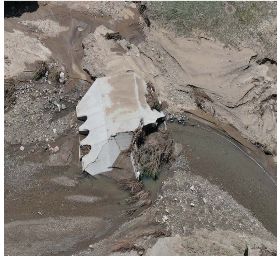
Photo 3. There are two culverts installed at the stream crossing. This appears to be inadequate as the prior cement culvert shown in the photo on the right had 3 large culverts.
