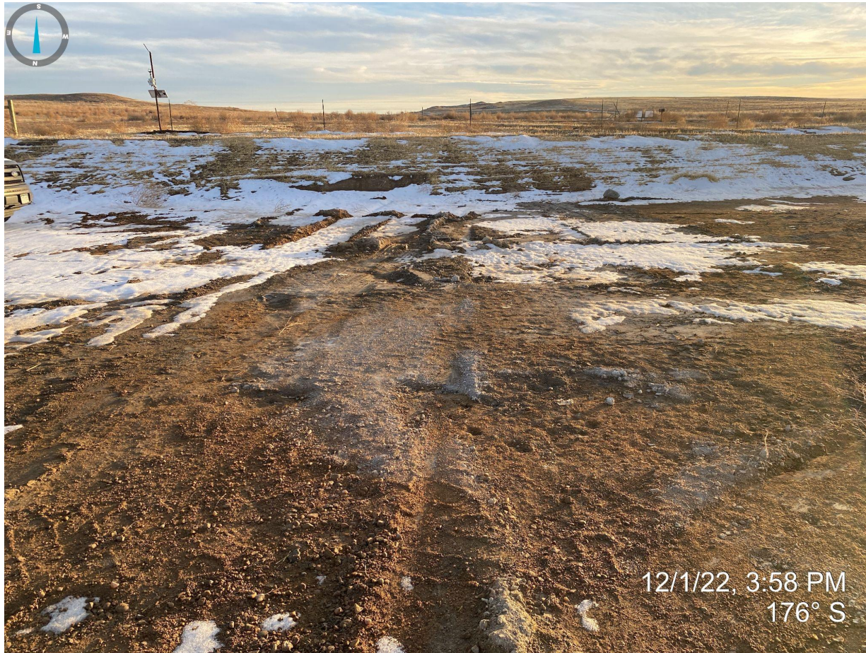
Photo 11. Facing south near the location entrance. Photo illustrates concrete debris/wash-out adjacent to interior ditch and berm. This is considered debris and needs to be removed.
