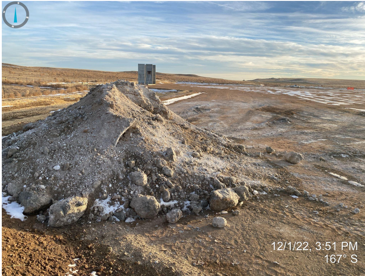
Photo 10. Facing south from the northeast corner of the pad. Photo shows a pile of concrete, without secondary containment, placed immediately adjacent to stormwater ditch and berm. This is considered debris and needs to be removed.
