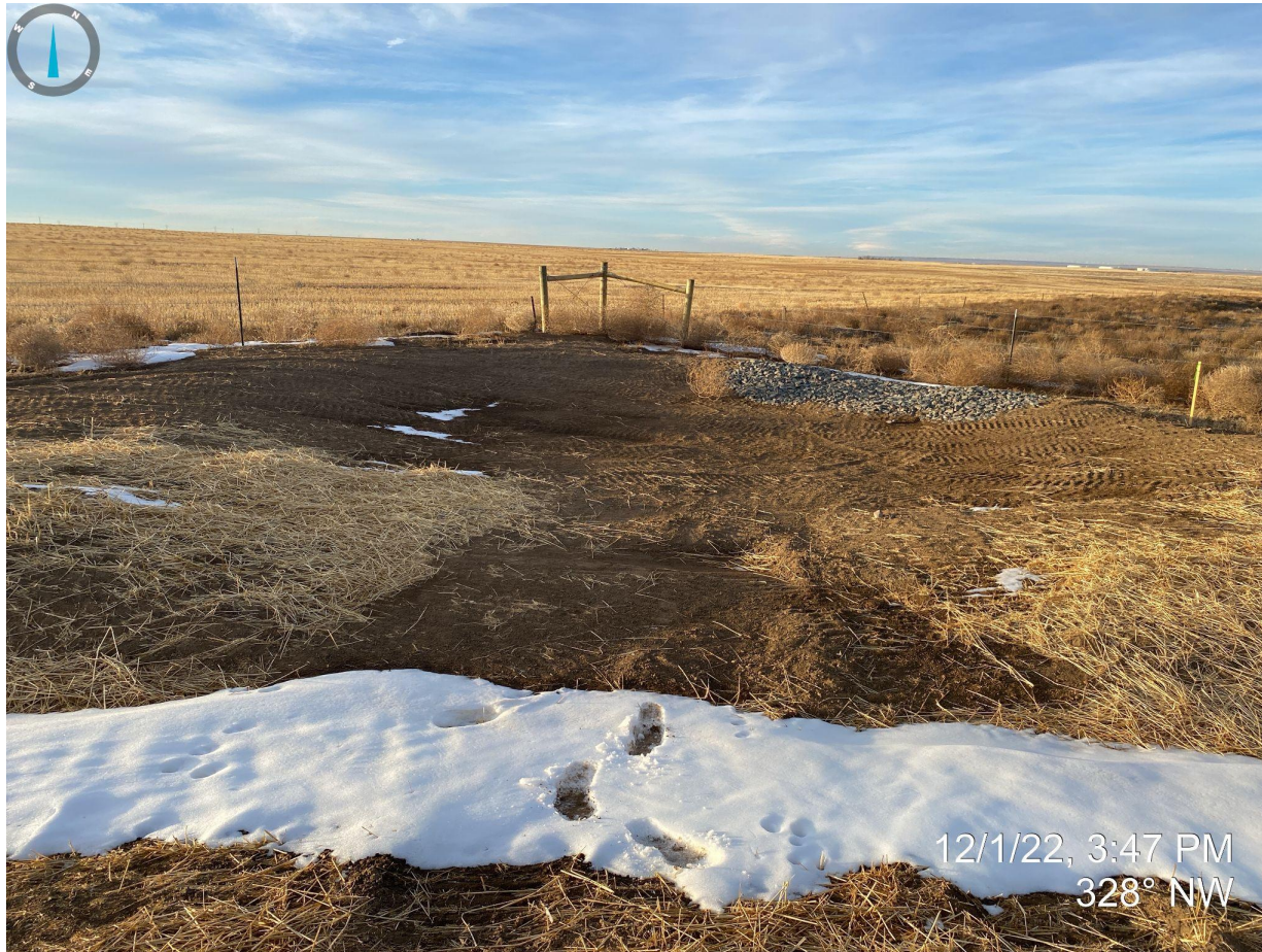
Photo 7. Facing northwest from the northwest corner of the location. Sediment trap appears inadequate in size to handle a 1-hour, 100-year stormwater event as per Weld County guidelines for stormwater management.
