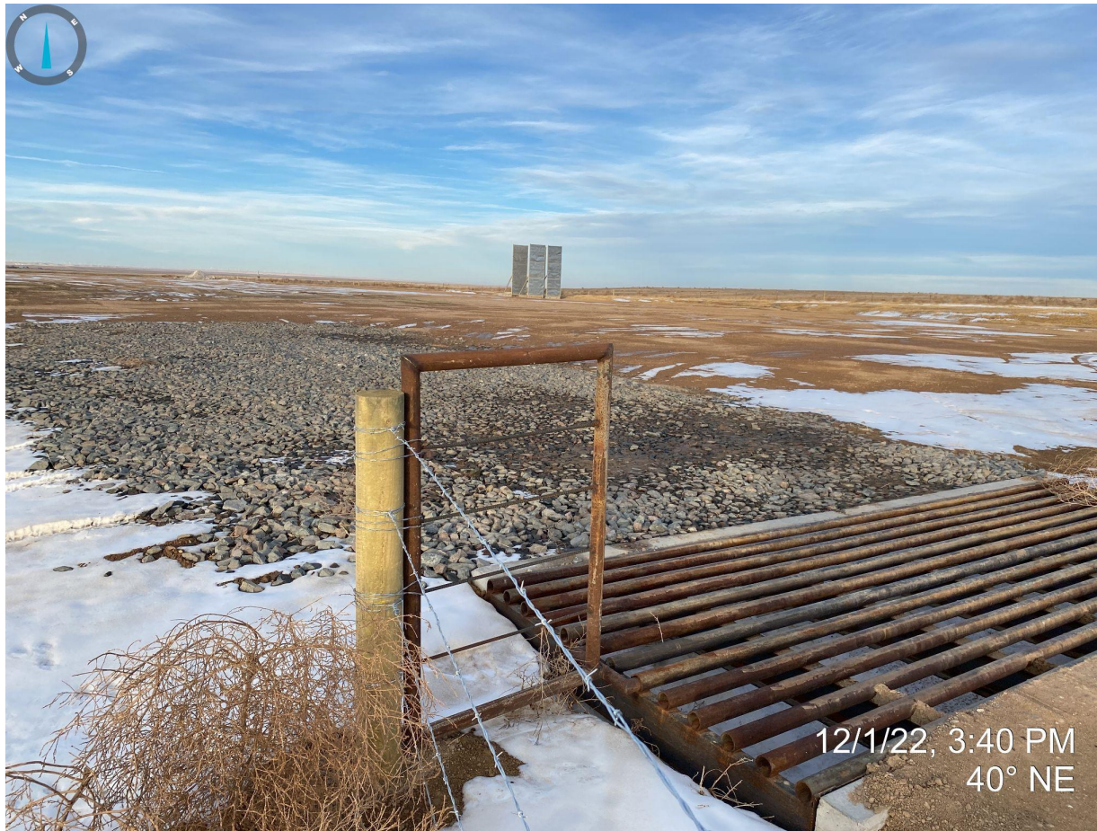
Photo 2. Facing northeast from entrance. Photo illustrates vehicle track out pad installed on location.
