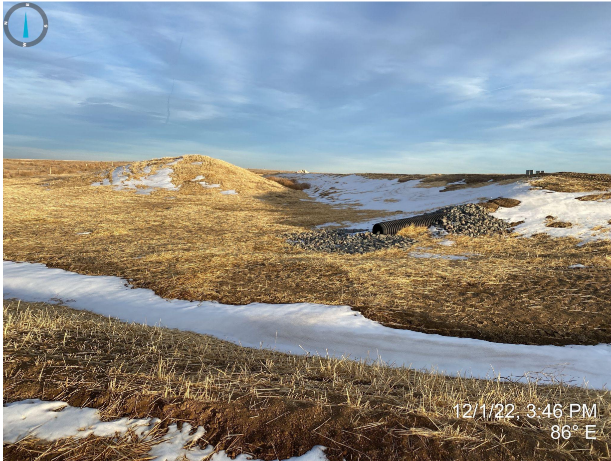
Photo 5. Facing east from the northwest corner of the location. Photo illustrates the topsoil stockpile has been temporarily stabilized with evidence of drill rows and crimped straw/mulch for long-term stabilization.
