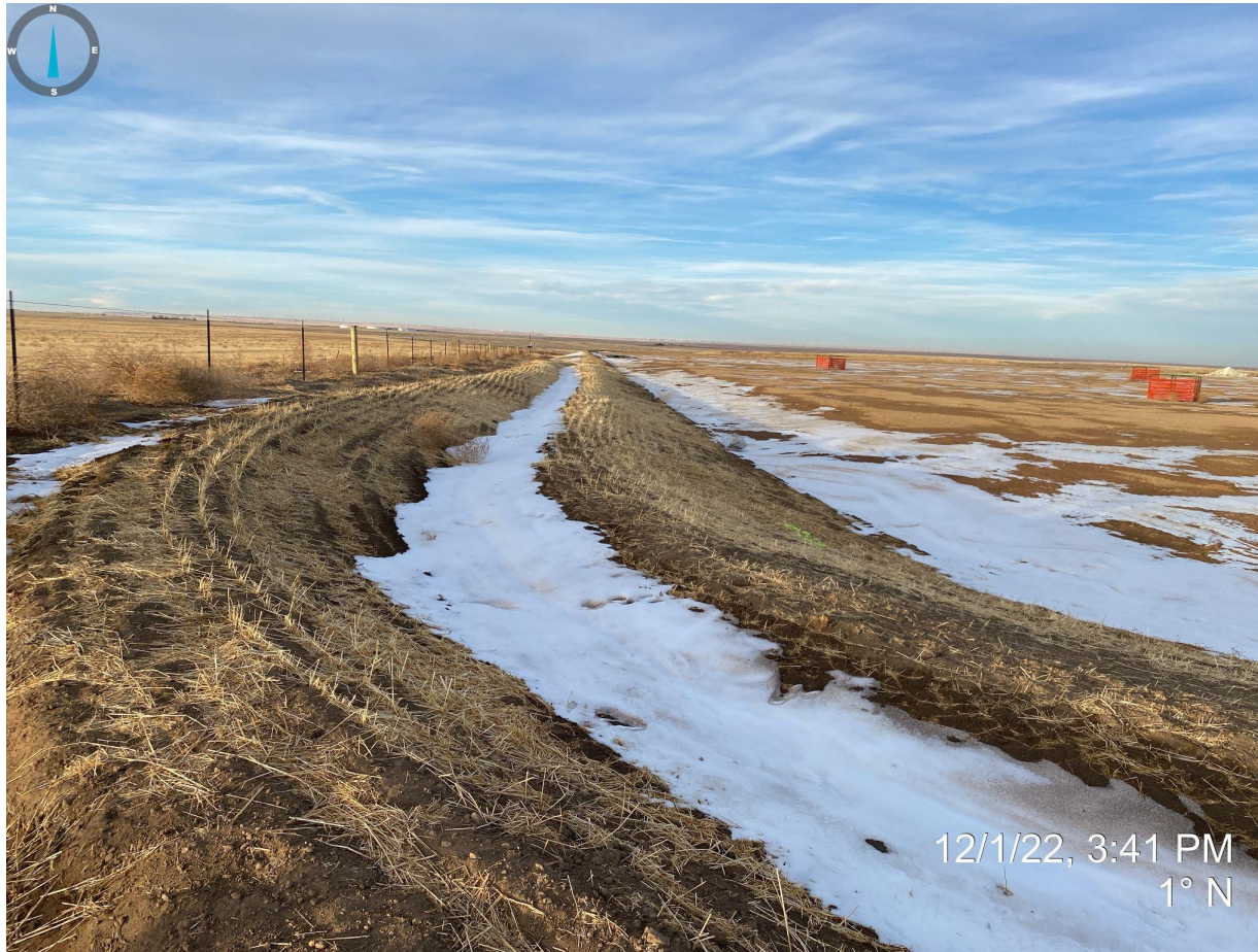
Photo 3. Taken from southwest corner, facing north. Photo illustrates the location has stormwater BMPs (e.g. ditch and berm) installed during the construction phase of the location. It appears the ditch and berm have been temporarily stabilized from wind and water erosion with evidence of drill rows and crimped mulch.
