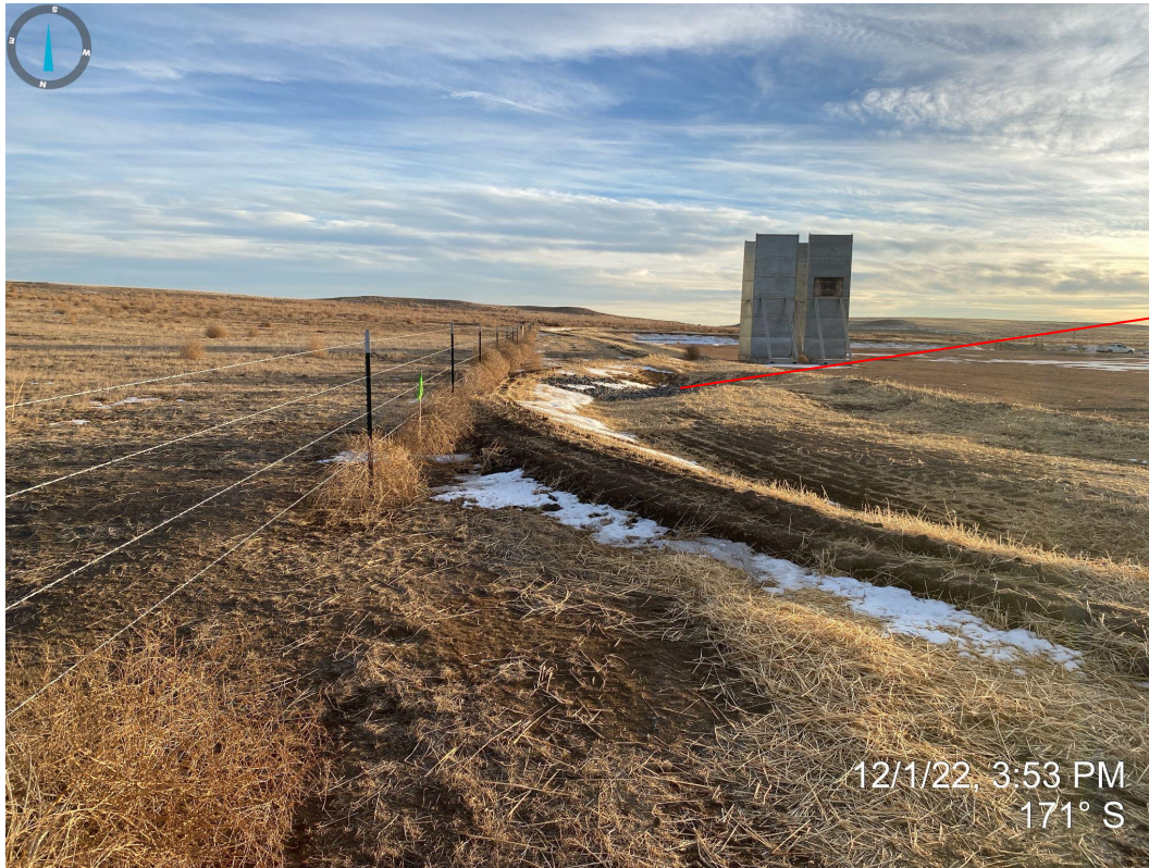
Photo 9. Facing south from the east portion of the location. Photo shows perimeter ditch and berm constructed with smaller sediment trap and outflow protection. Tumbleweeds gathered alongside of perimeter fence are considered debris and need to be removed.
