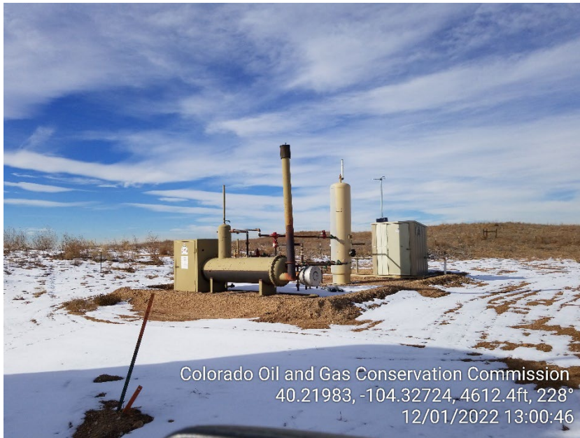
Photo 3 – Separator and Gas Meter
