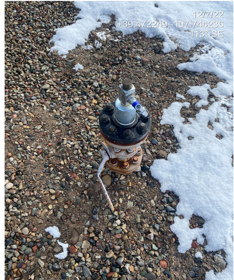
Photo 2. Photo shows production areas. Note improperly abandoned flowline riser not locked out/tagged out.
