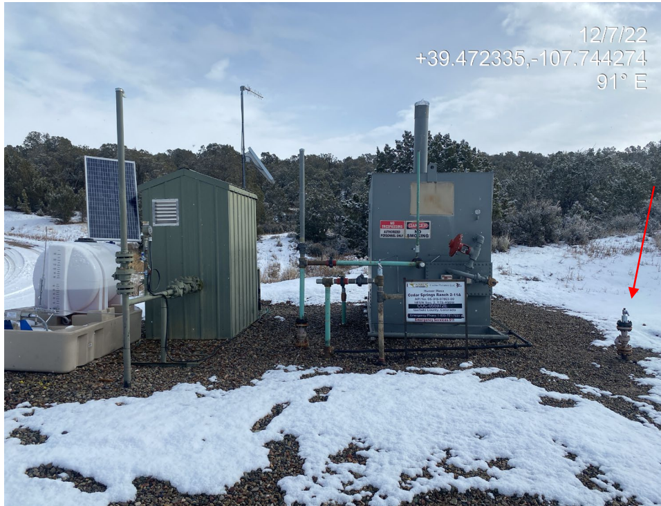
Photo 2. Photo shows production areas. Note improperly abandoned flowline riser not locked out/tagged out.
