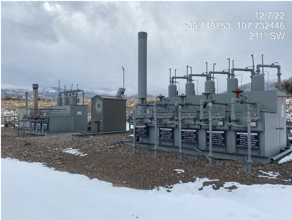
Photo 2. Photos show production areas. Caps have been installed on separator lines.
