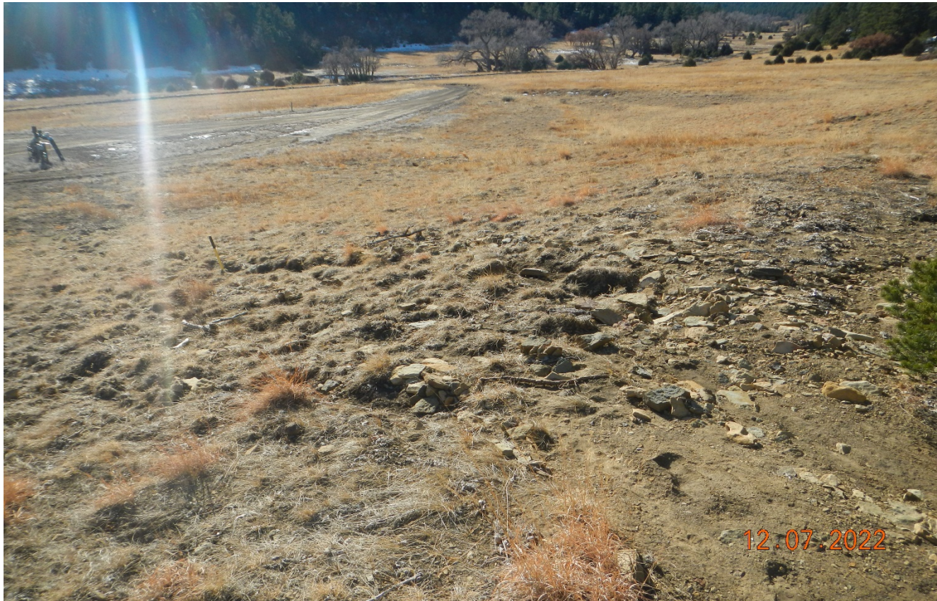
Photo 7. Facing south toward the run-on ditch which is filled in with sediment causing erosion of the cut slope. Previous corrective action is not completed.
