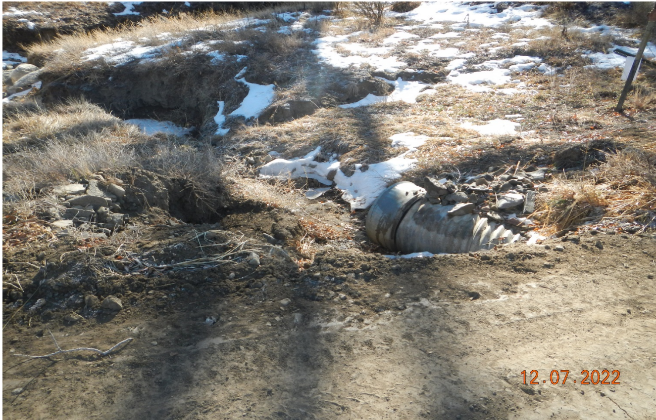
Photo 3. The next culvert along the road is also eroded at the culvert outlet with no outlet protection. Previous corrective action was not completed.
