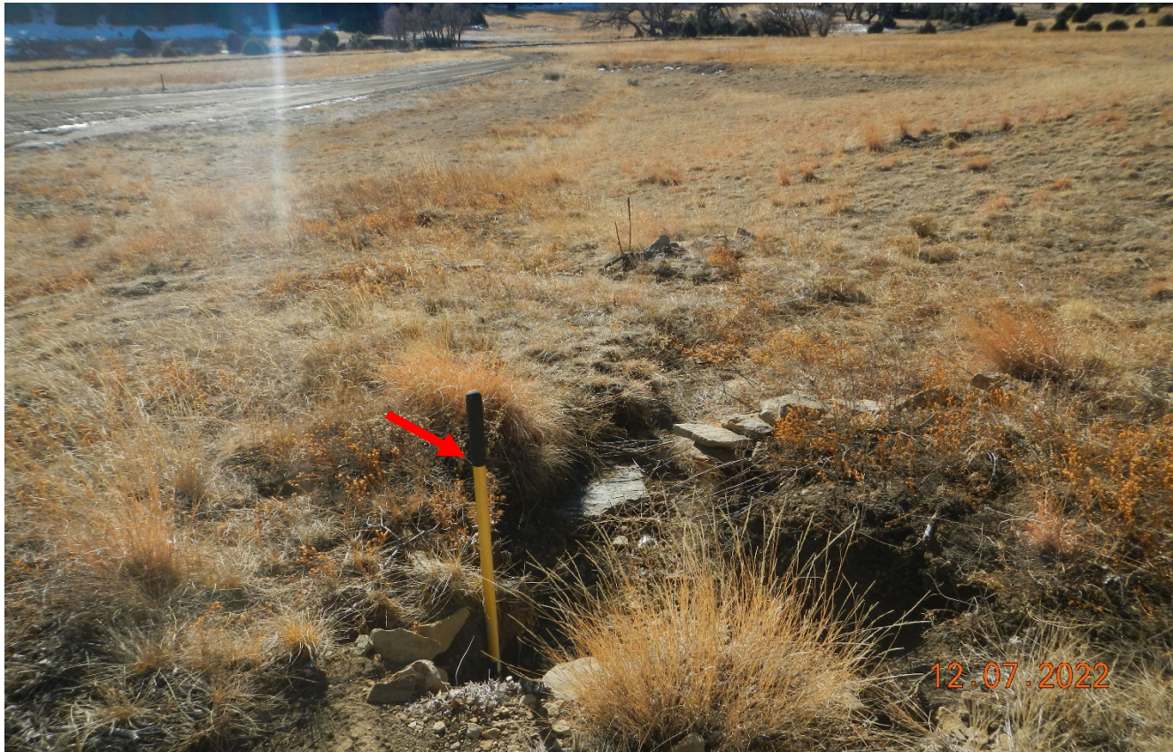
Photo 8. There are additional erosion channels along the south side of the location. Previous corrective action is not completed. Red arrow points to 4.5 ft. shovel placed in the erosion channel.
