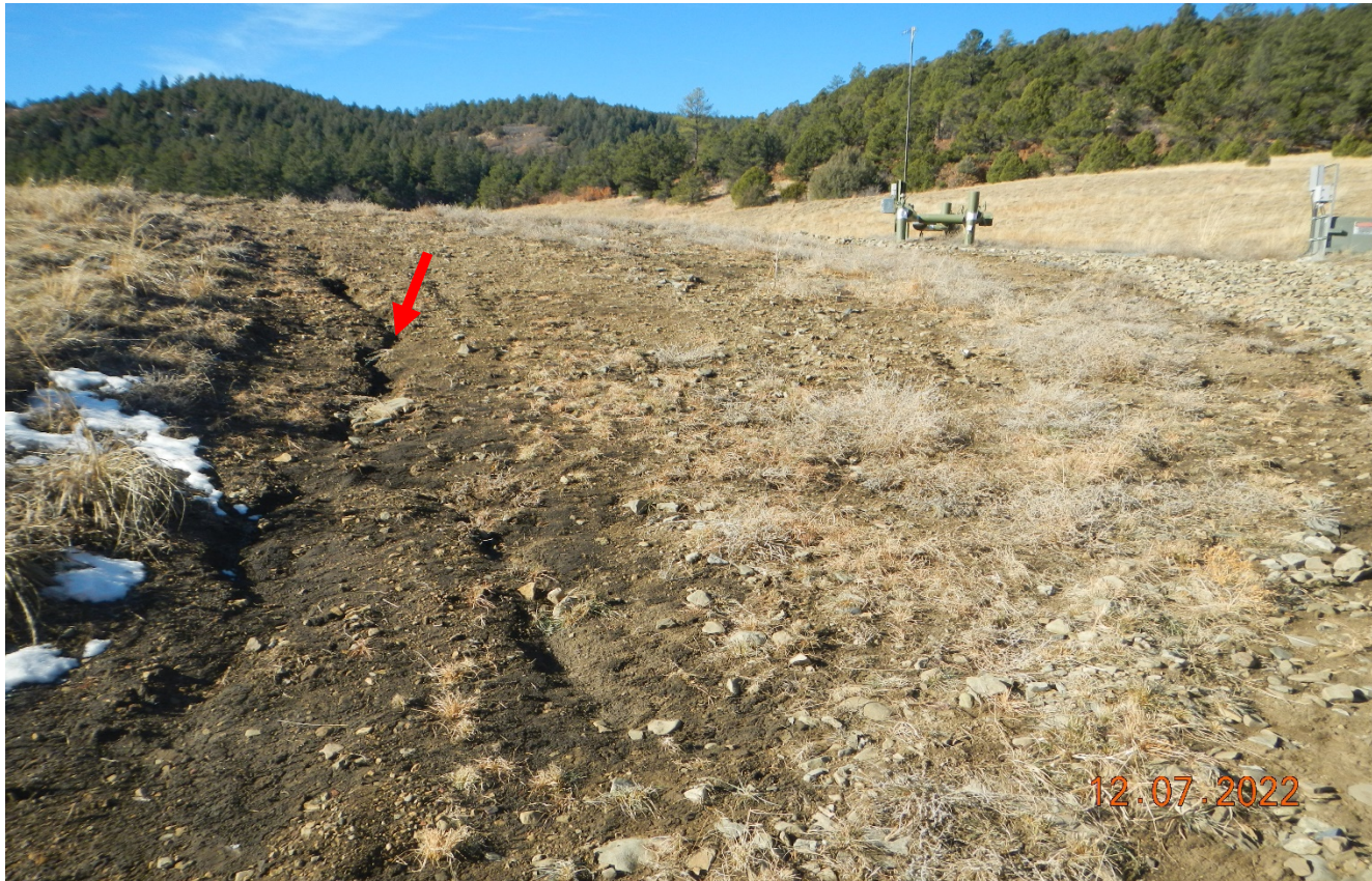
Photo 4. Facing southwest at the location. There is erosion occurring off the northeast side of the location. Additional BMP's need to be installed in this area.
