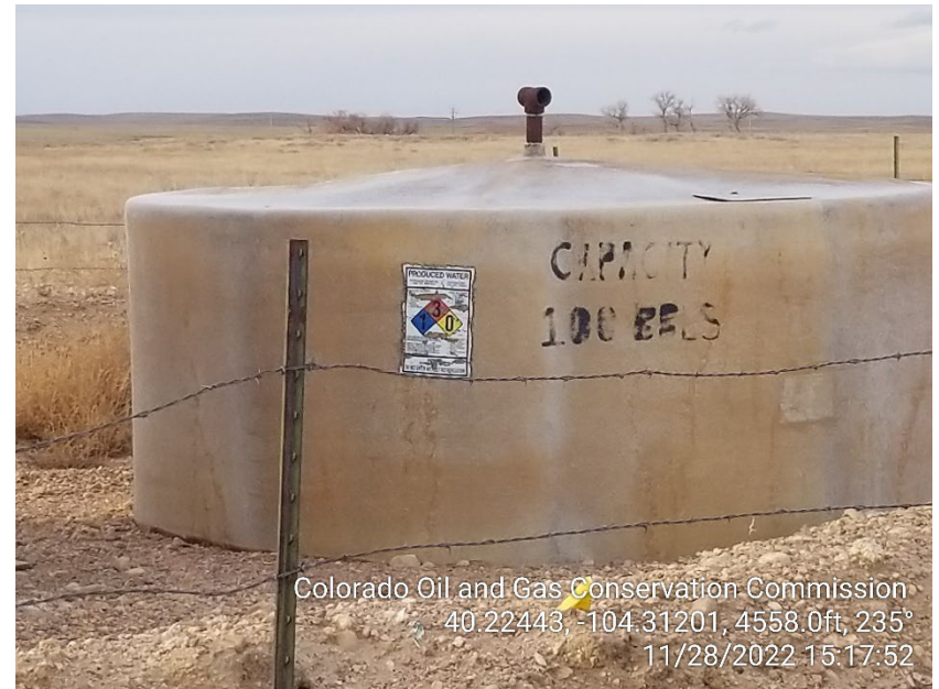
Photo 2 – Produced Water Tank
