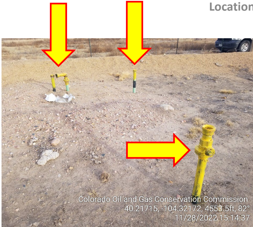
Photo 5 – Unmarked Risers
