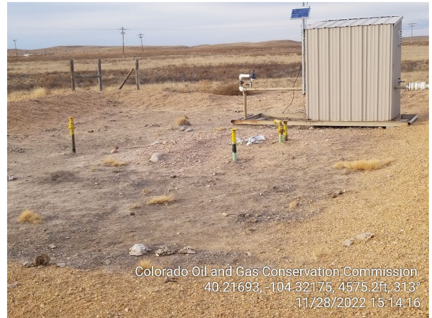
Photo 4 – Unmarked Risers
