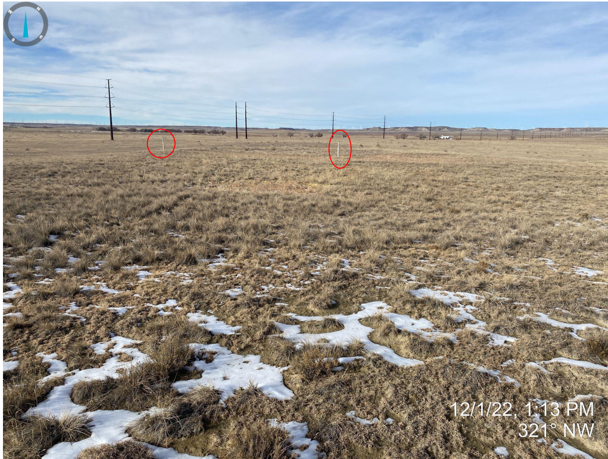
Photo 2. Taken from the southern portion of the well location, facing north. Photo illustrates the location has been reclaimed with presence of desirable vegetation (e.g. buffalo grass, sand drop seed, etc). The red outlined pipeline markers need to be removed.
