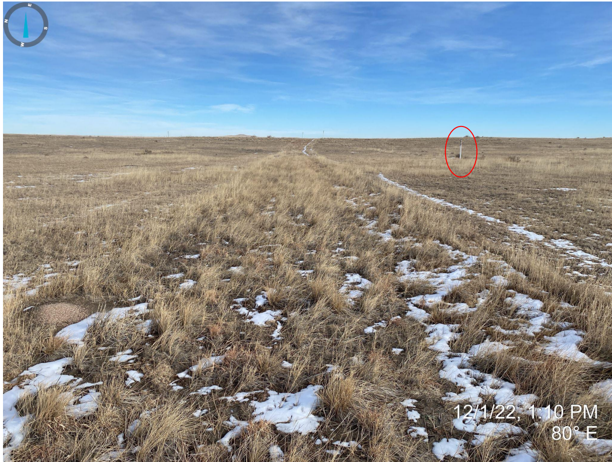
Photo 1. Taken north of the tank battery, facing east. Photo illustrates that the access road has been reclaimed and revegetated with desirable species. Red outline indicates pipeline markers that need to be removed.
