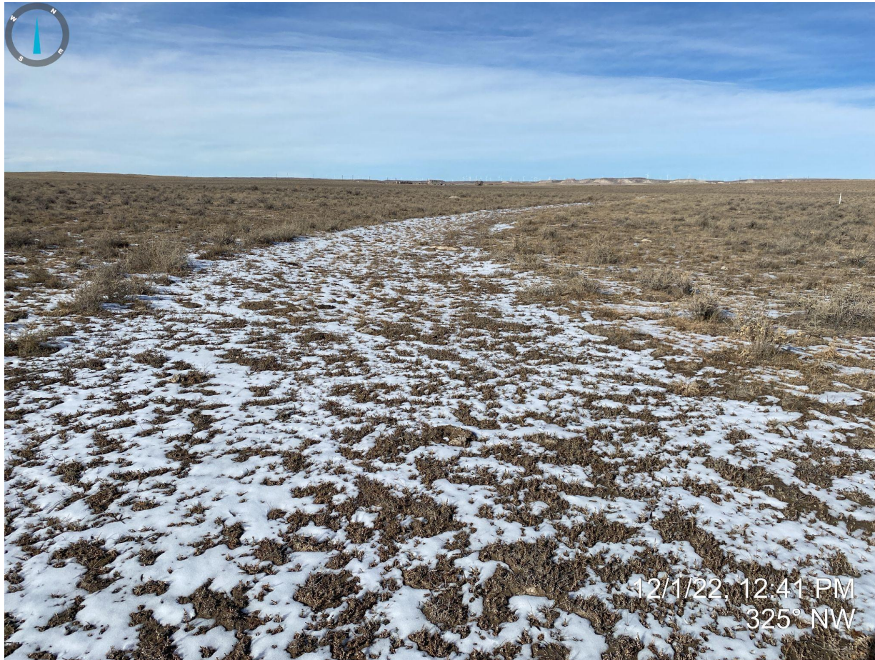
Photo 1. Taken from the southern access road entrance, facing northwest. Photo illustrates the access road has not revegetated and does not meet 1004 reclamation standards. Undesirable vegetation (e.g. russian thistle and kochia) was observed throughout the majority of the former access road.
