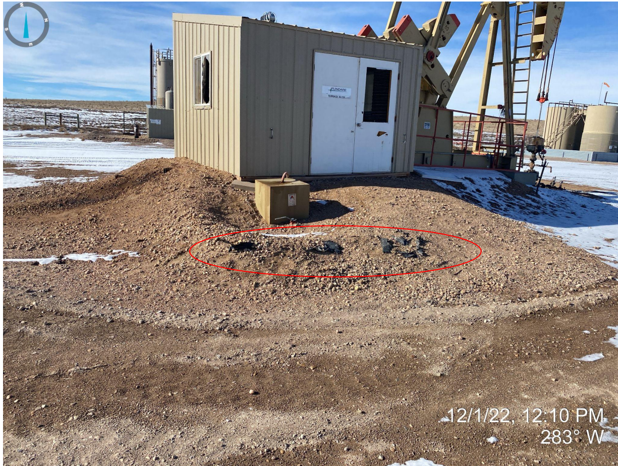
Photo 2. Facing west at pump jack. Photo illustrates the berm around the condensate tank is inadequate as the eastern berm wall is degrading/eroded away.
