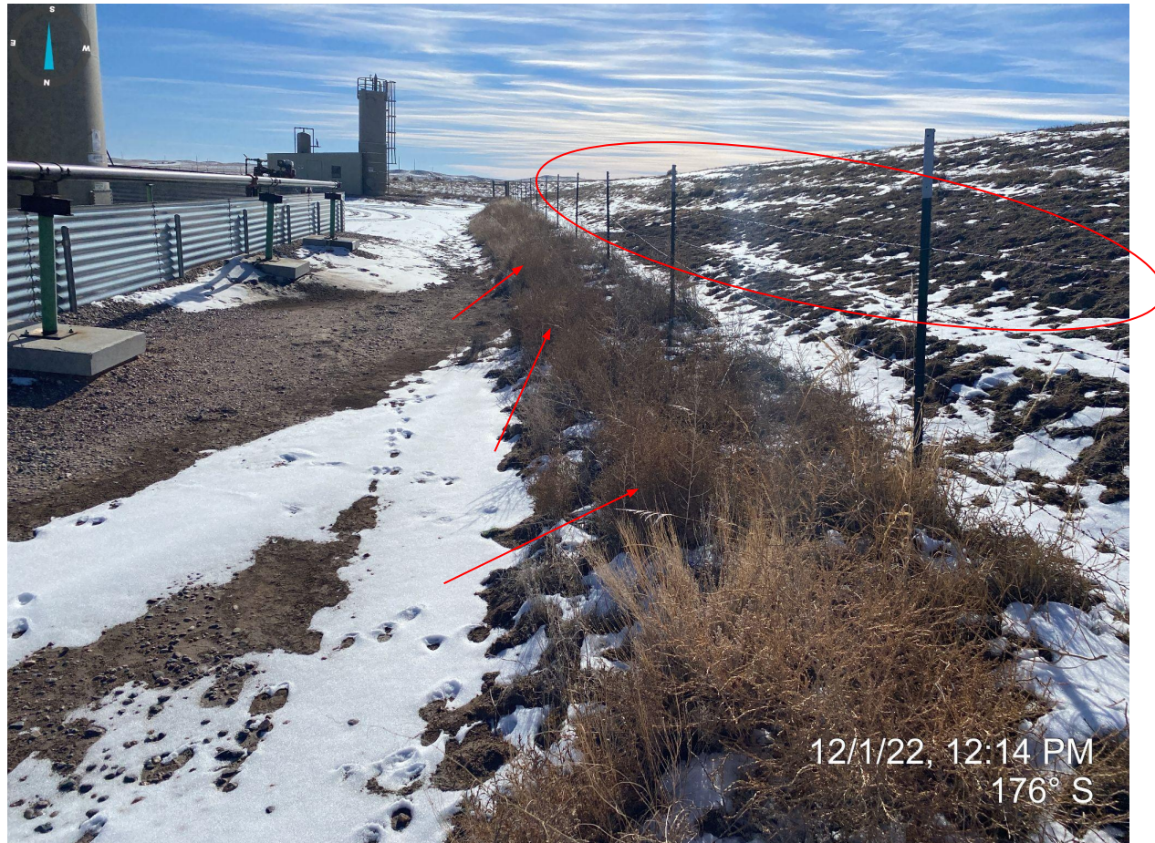
Photo 6. Taken from the western portion of the location, facing south. Photo illustrates evidence of undesirable vegetation (e.g. russian thistle and kochia) and also shows areas of bare soil within the cut slope for the location.
