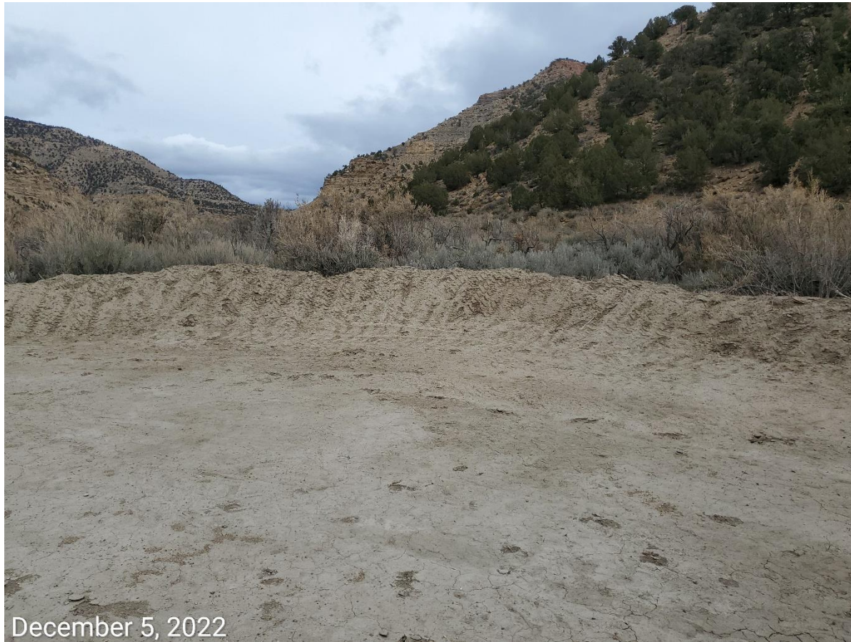
Photo 5: Photo show tracking implemented at slopes on the northeast end of the Location.
