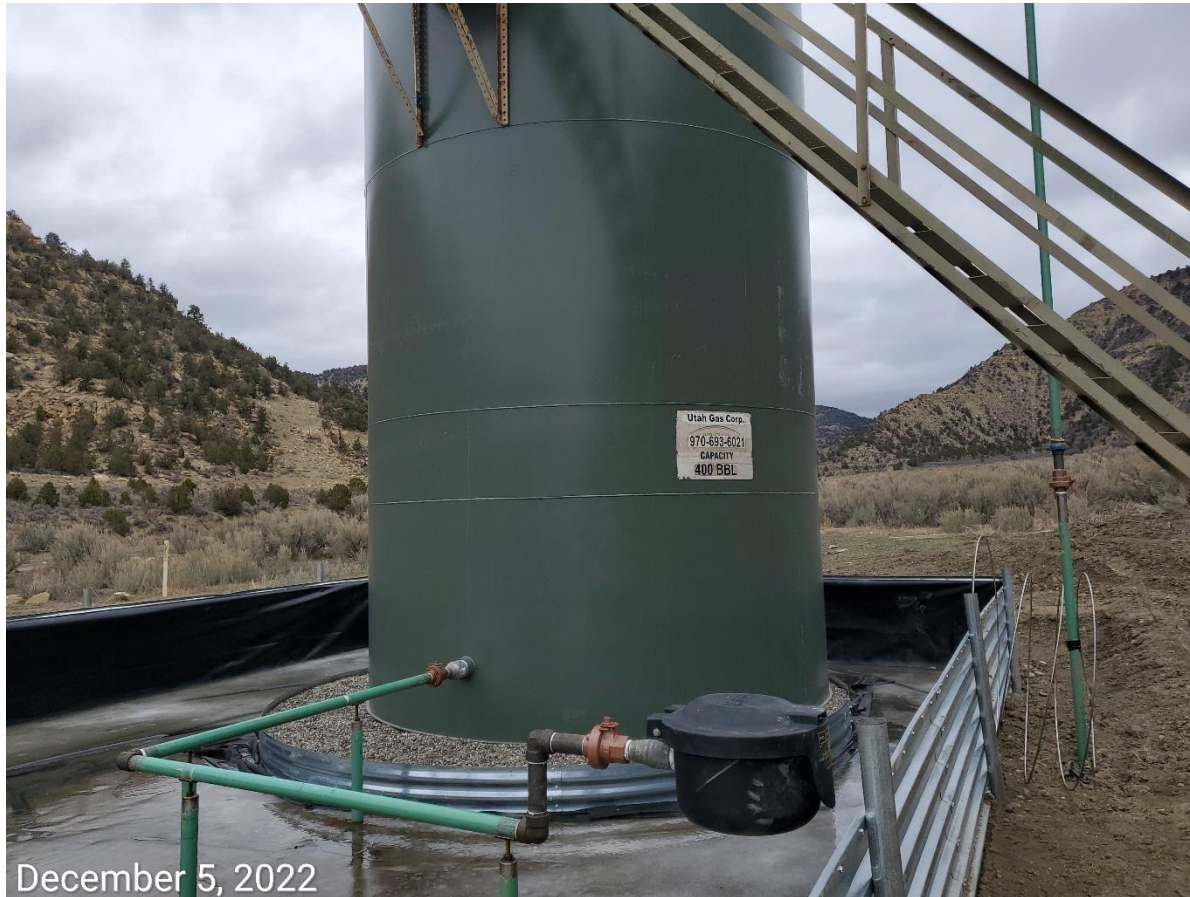
Photo 5: Photo shows recently installed tank battery. Label on tank missing required contents information.
