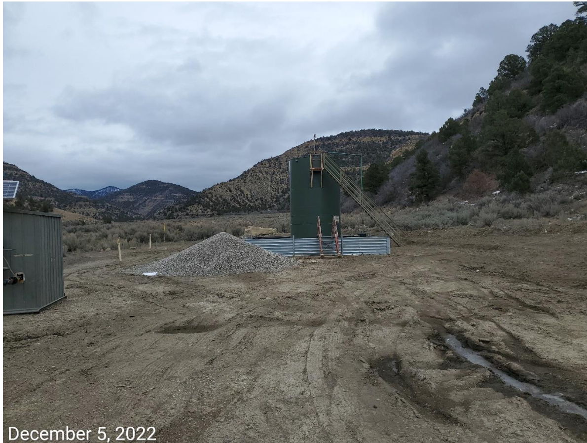
Photo 8: Photo shows signage missing from tank battery. Photo also shows stockpiled gravel material on the Location.
