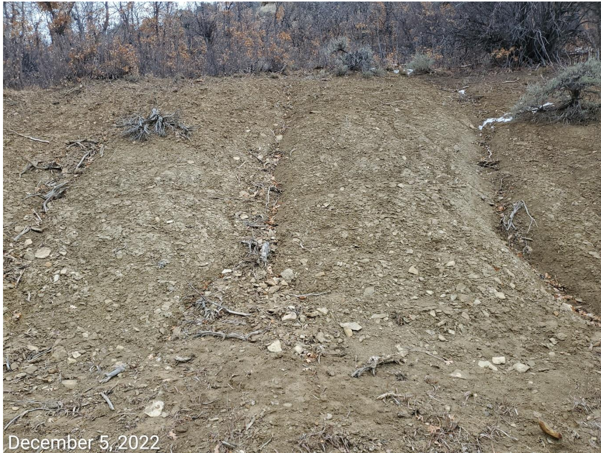
Photo 6: Photo taken from the northeast end of the Location. Photo shows cut slope remaining. Photo also shows erosion degradation along the slopes.
