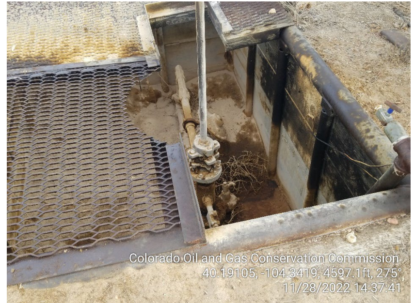
Photo 4 – Stained Soil at Wellhead
