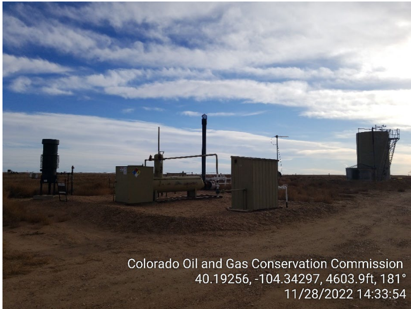
Photo 1 – Separator, ECD and Gas Meter
