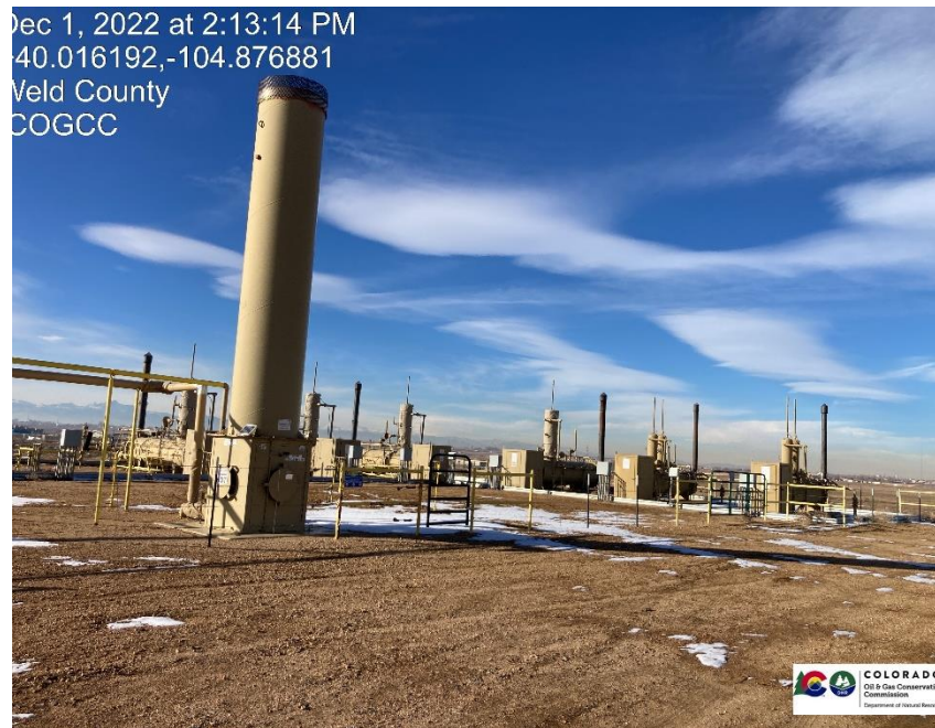
Pic 4 ECD, separators.
