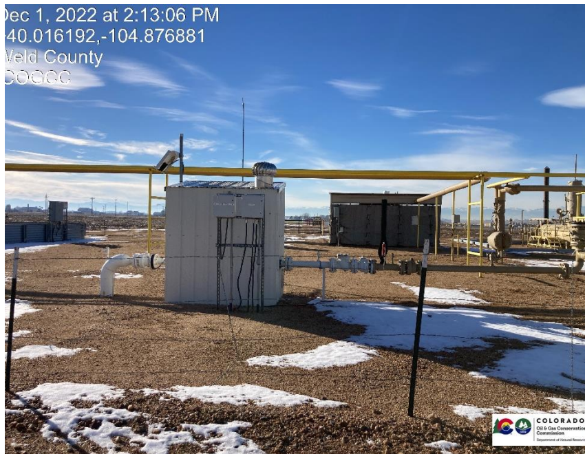
Pic 3 gas meter run, VRU
