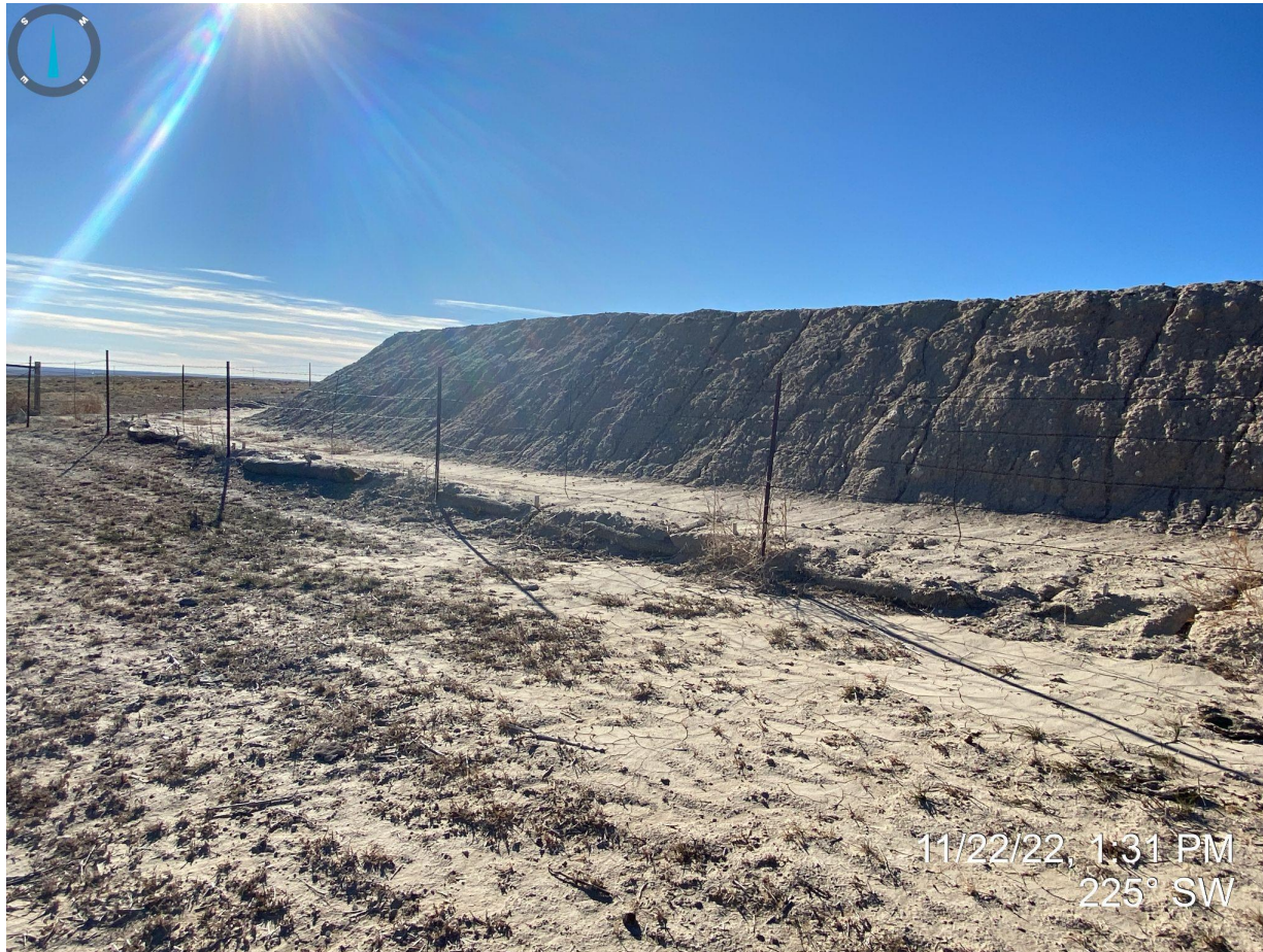
Photo 14. Taken east of the pit, facing southwest. Photo illustrates that the pit walls are unstabilized as evidenced by rill erosion and there are no apparent stormwater BMPs to prevent sediment laden stormwater from exiting off location. Areas of bare soil in foreground are a result of stormwater exiting off location and impacts of salt kill.
