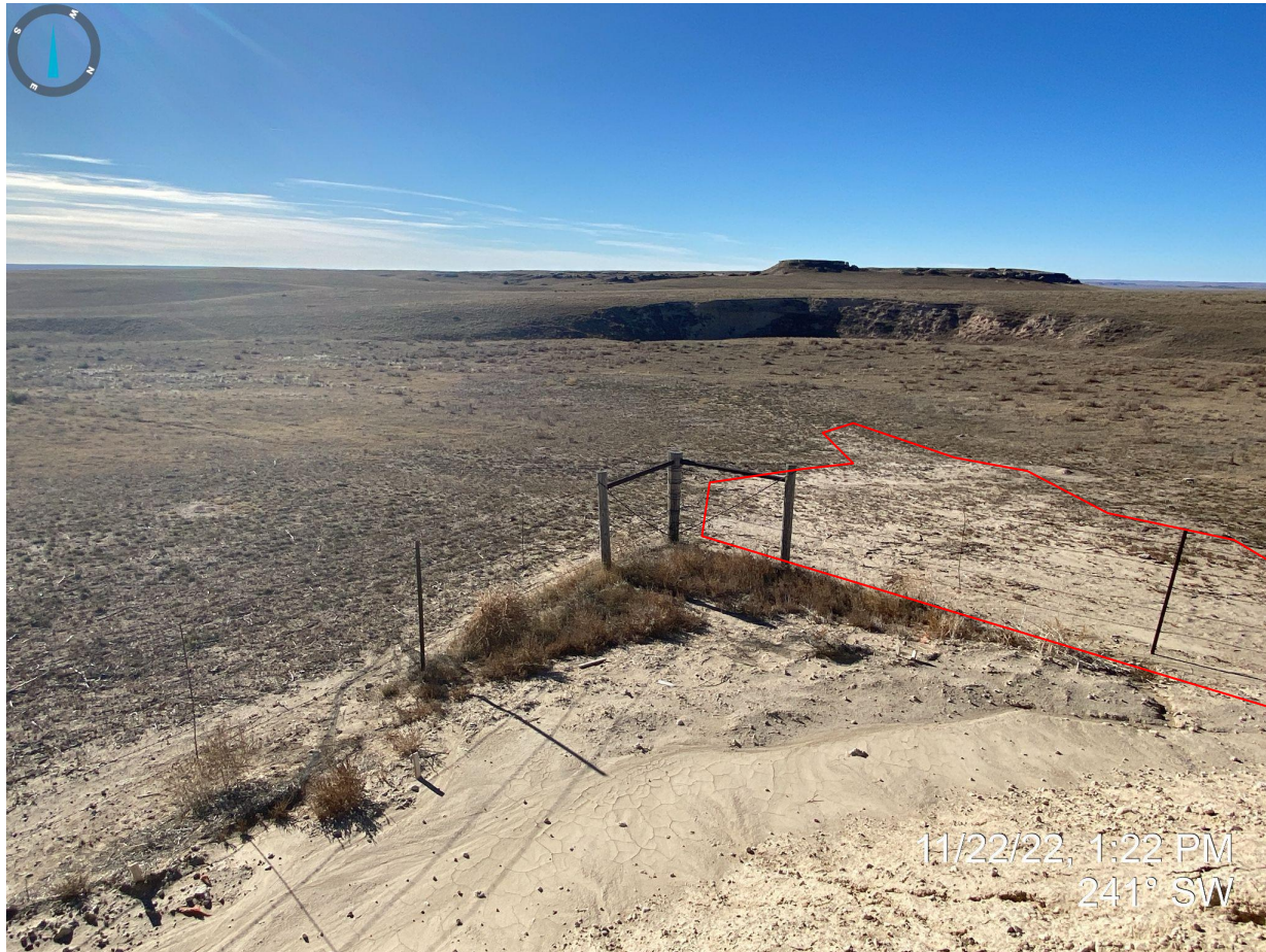
Photo 19. Taken from the southwest pit wall, facing southwest. Photo illustrates that no stormwater BMPs appear to be implemented and that sediment laden stormwater has exited off location, outlined in red.
