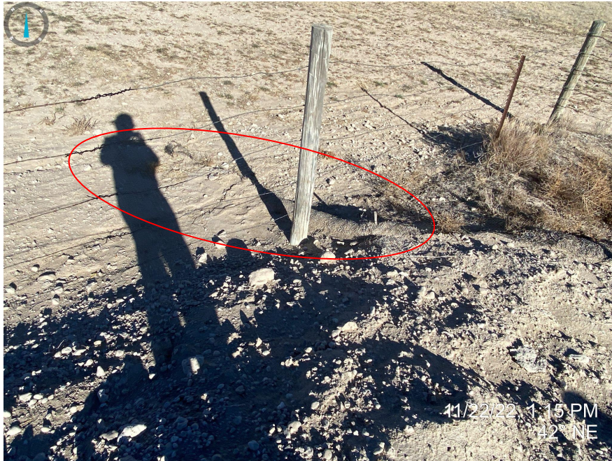
Photo 12. Taken from the northeast pit wall, facing northeast. Photo illustrates a buried straw wattle (left photo); and the right photo shows rill erosion occurring on the pit walls. It does not appear there are any stormwater BMPs to prevent sediment laden stormwater from exiting off location, outlined in red.
