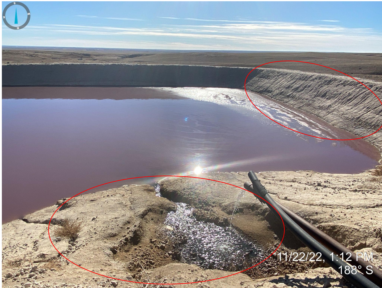
Photo 6. Taken from the northern wall of the pit, facing south. Photo illustrates rill and gully erosion on the pit walls, outlined in red.
