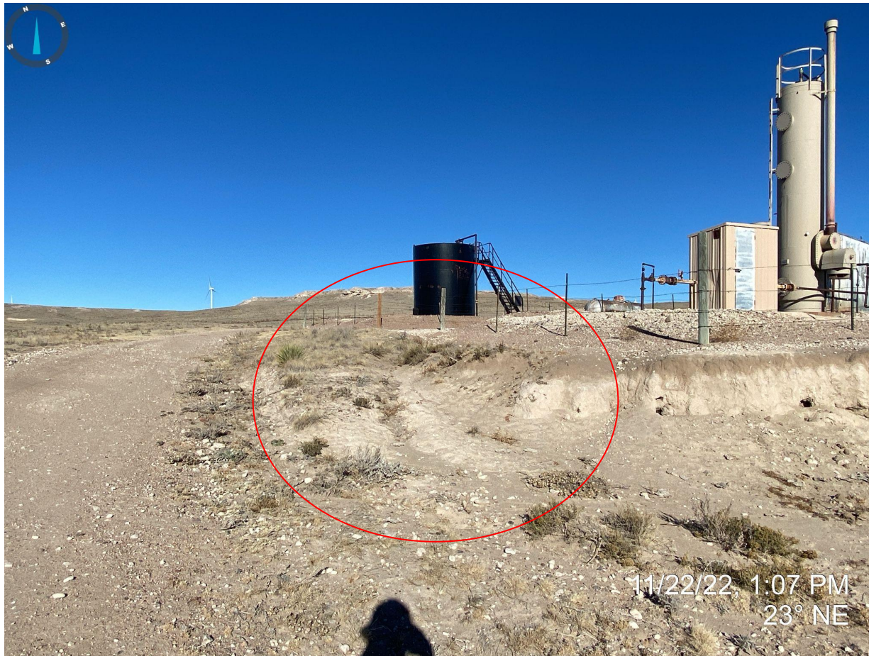
Photo 5. Taken from the northern portion of the location, facing northeast. Photo illustrates gully erosion that has not been stabilized and/or had stormwater BMPs implemented; this has been addressed in prior inspections.
