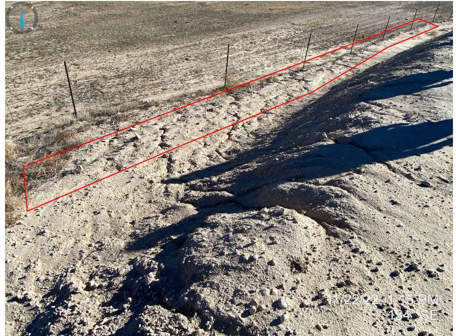
Photo 12. Taken from the northeast pit wall, facing northeast. Photo illustrates a buried straw wattle (left photo); and the right photo shows rill erosion occurring on the pit walls. It does not appear there are any stormwater BMPs to prevent sediment laden stormwater from exiting off location, outlined in red.
