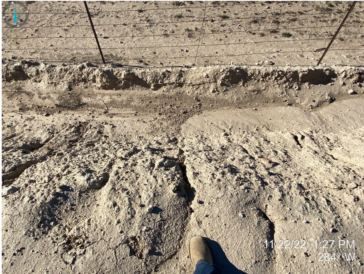
Photo 21. Taken from the western pit wall, facing west. Photo illustrates the unstabilized pit walls and evidence of rill erosion.
