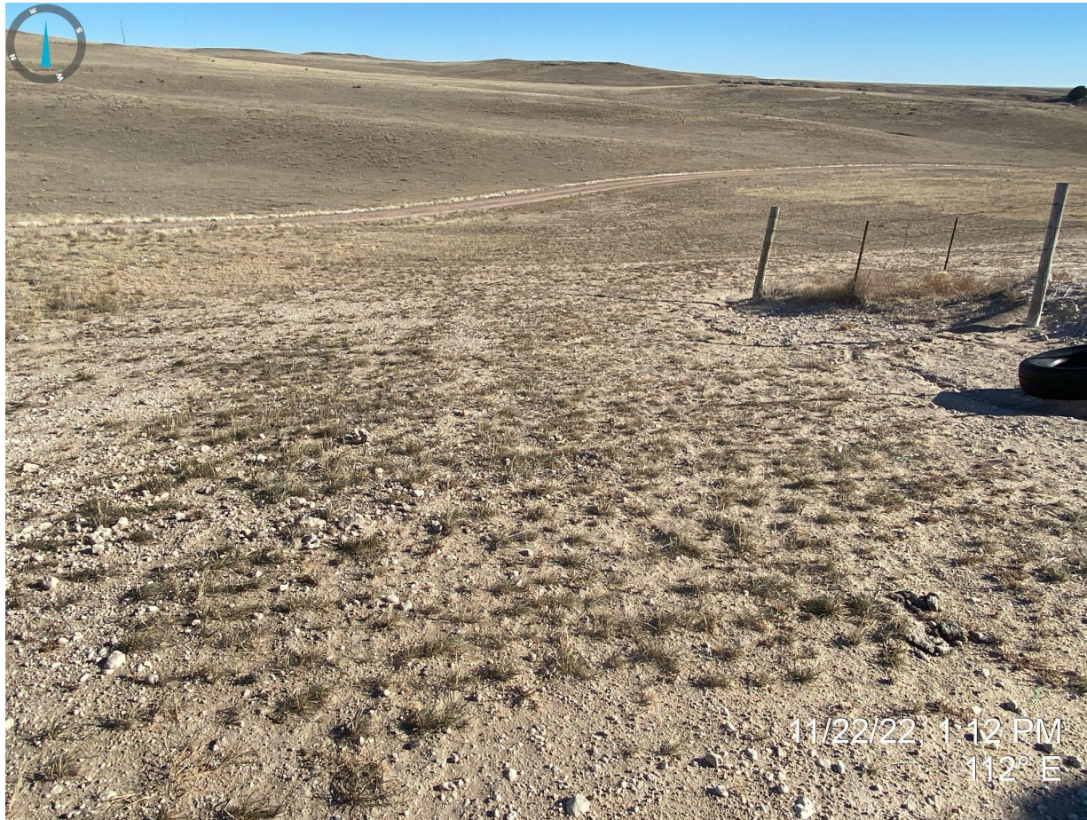
Photo 10. Taken from the northeast corner of the pit, facing east. Photo illustrates that reclamation efforts don't appear to be achieving reclamation standards as vegetation is sparse and bare soil is evident. Additionally, it does not appear that are any stormwater BMPs to prevent erosion from occurring.
