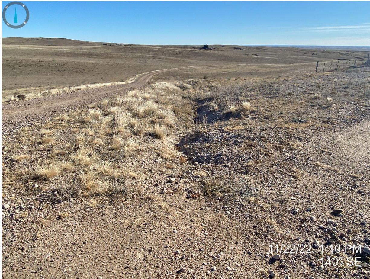
Photo 9. Taken from the eastern portion of the location, facing southeast. Photo illustrates gully erosion that has not been repaired and stabilized, and does not have any evidence of stormwater BMPs to prevent further off-site sediment transport and degradation to adjacent areas.
