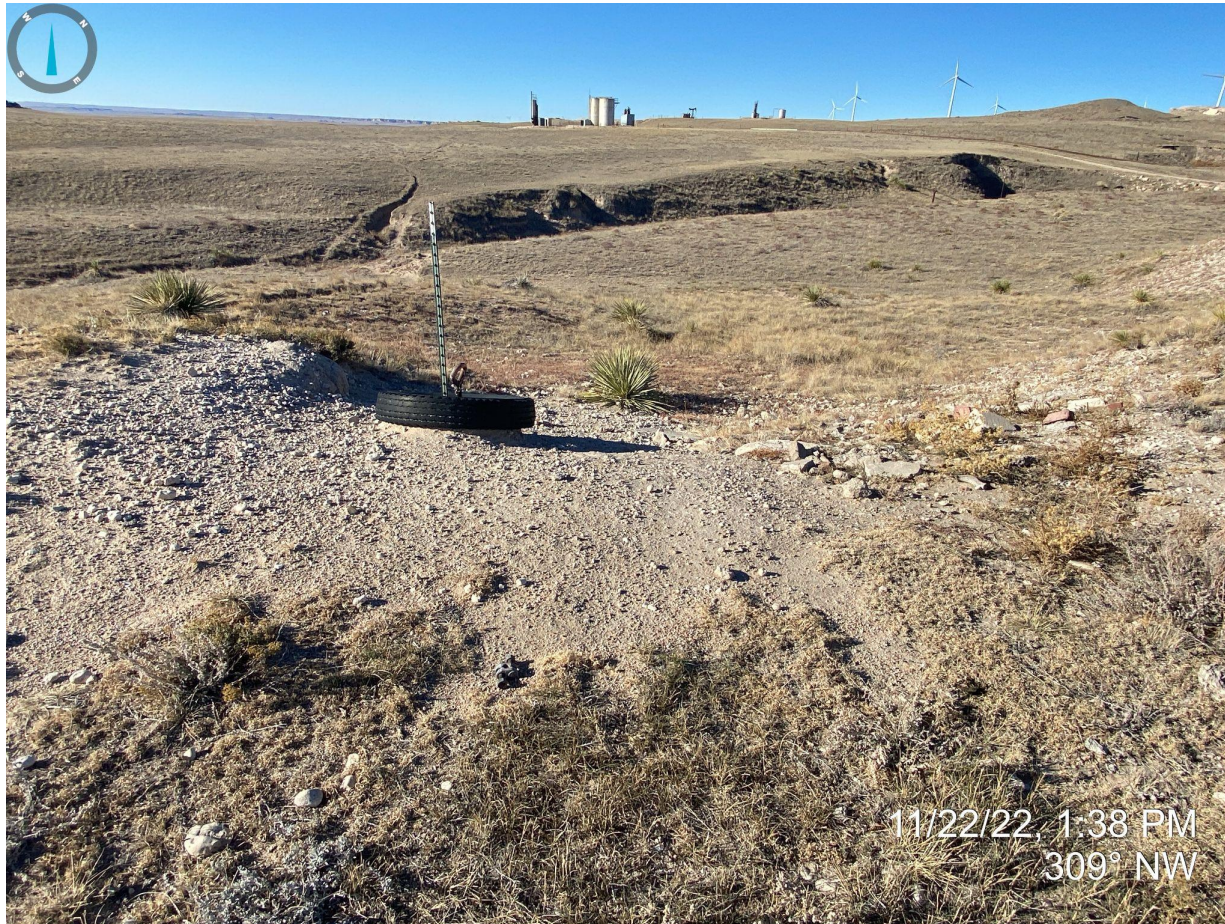
Photo 23. Taken from the northwestern portion of the location, facing northwest. Photo illustrates erosion occurring around one of the buried guy line anchors. This area needs to be stabilized with BMPs from wind and water erosion to prevent off-site degradation and sediment migration.
