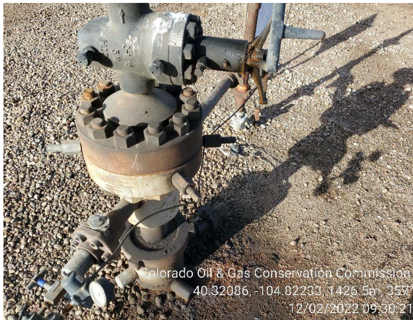
Master valve leak and stained soil
