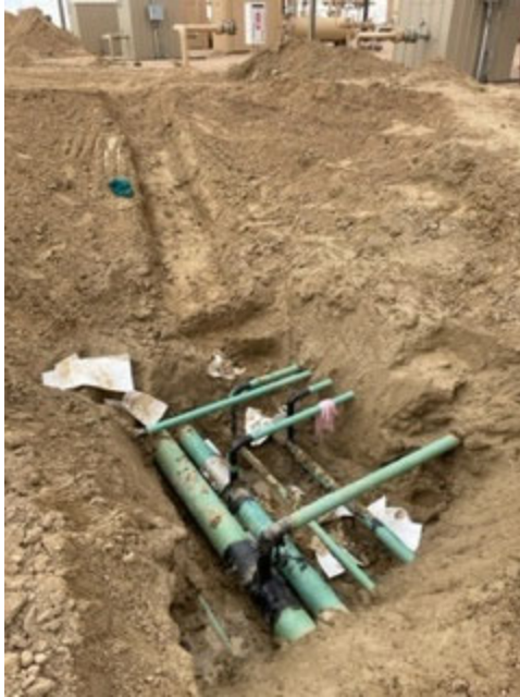
7 – Wells Ranch AE20 compromised flowline location within west excavation extent
