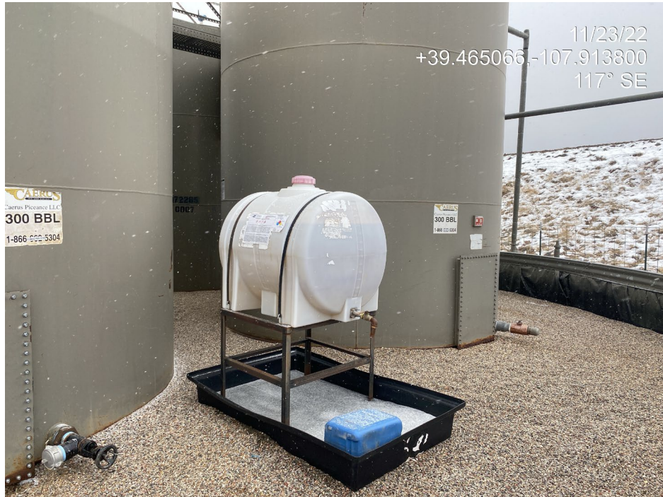
Photo 3. Photos show two secondary containment tanks lacking wildlife protection BMPs.
