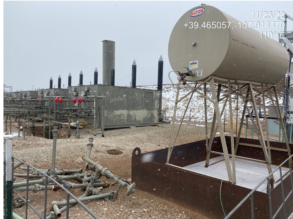
Photo 3. Photos show two secondary containment tanks lacking wildlife protection BMPs.
