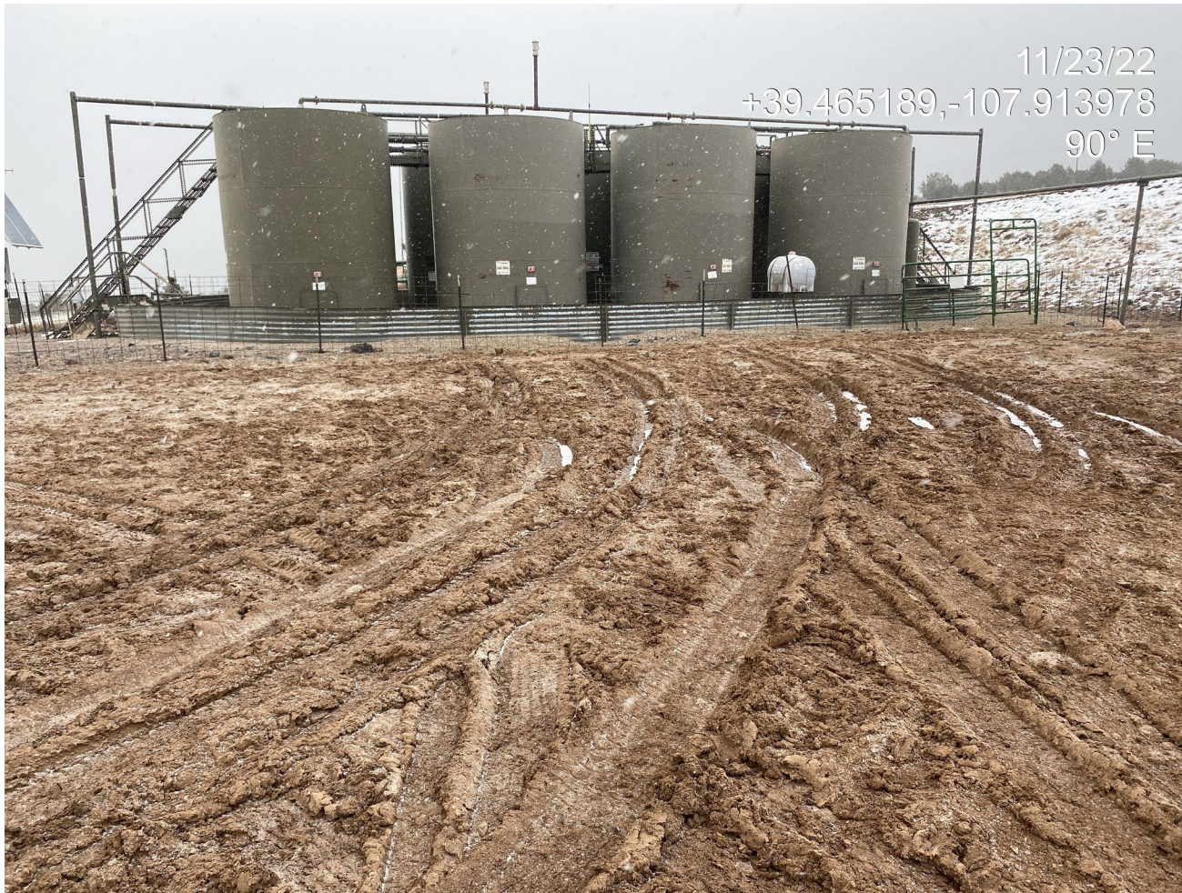
Photo 8. Photo shows degradation to the pad surface.
