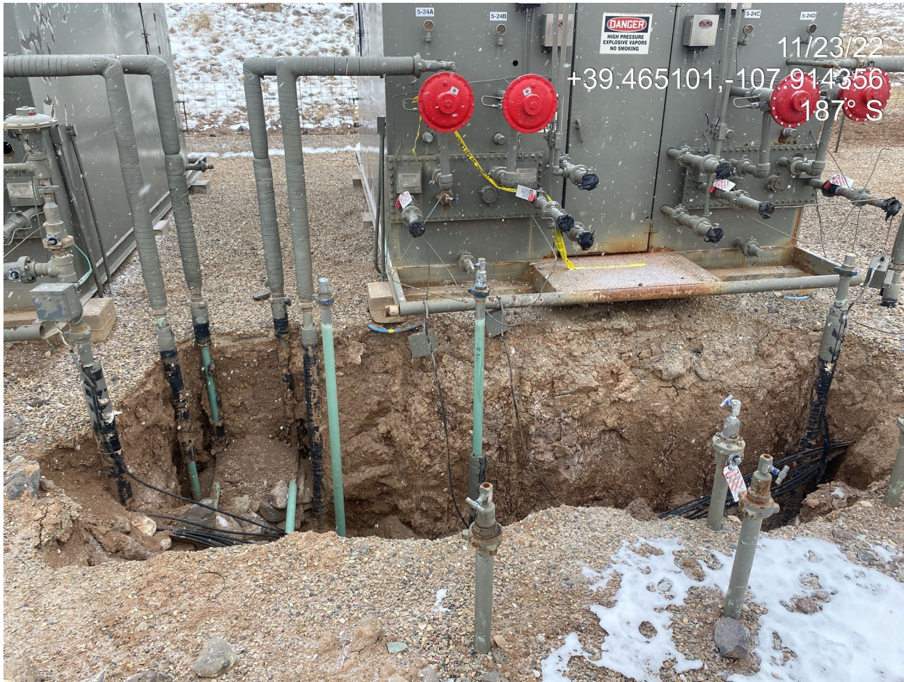
Photo 4. Photo taken from the south shows an excavation at the separators lacks protections to prevent personnel from entering or falling into the trench.
