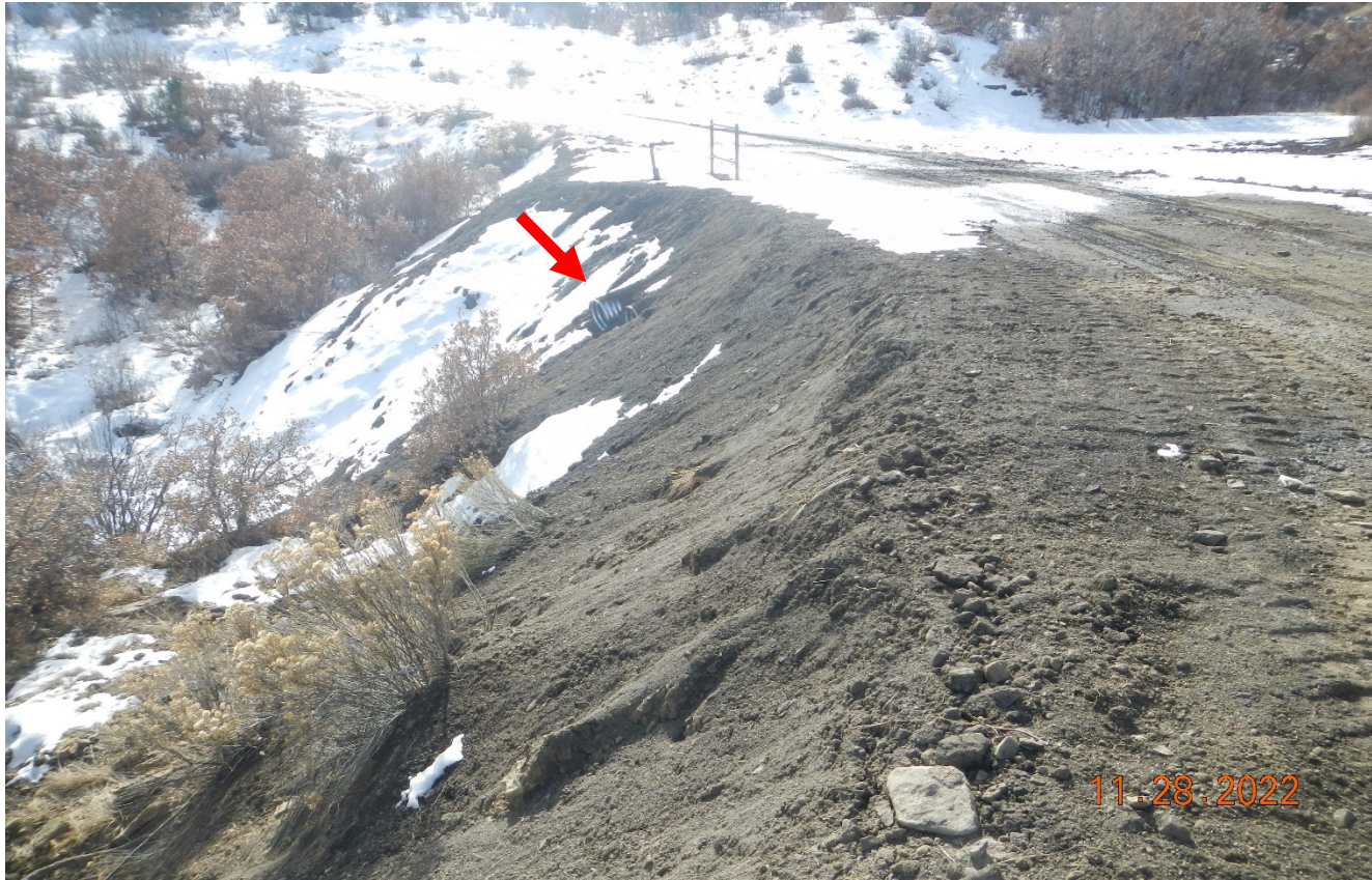
Photo 2. The eroded area of the road was repaired however, loose soils are not stabilized and will erode. There is no outlet protection installed at the culvert shown at red arrow.
