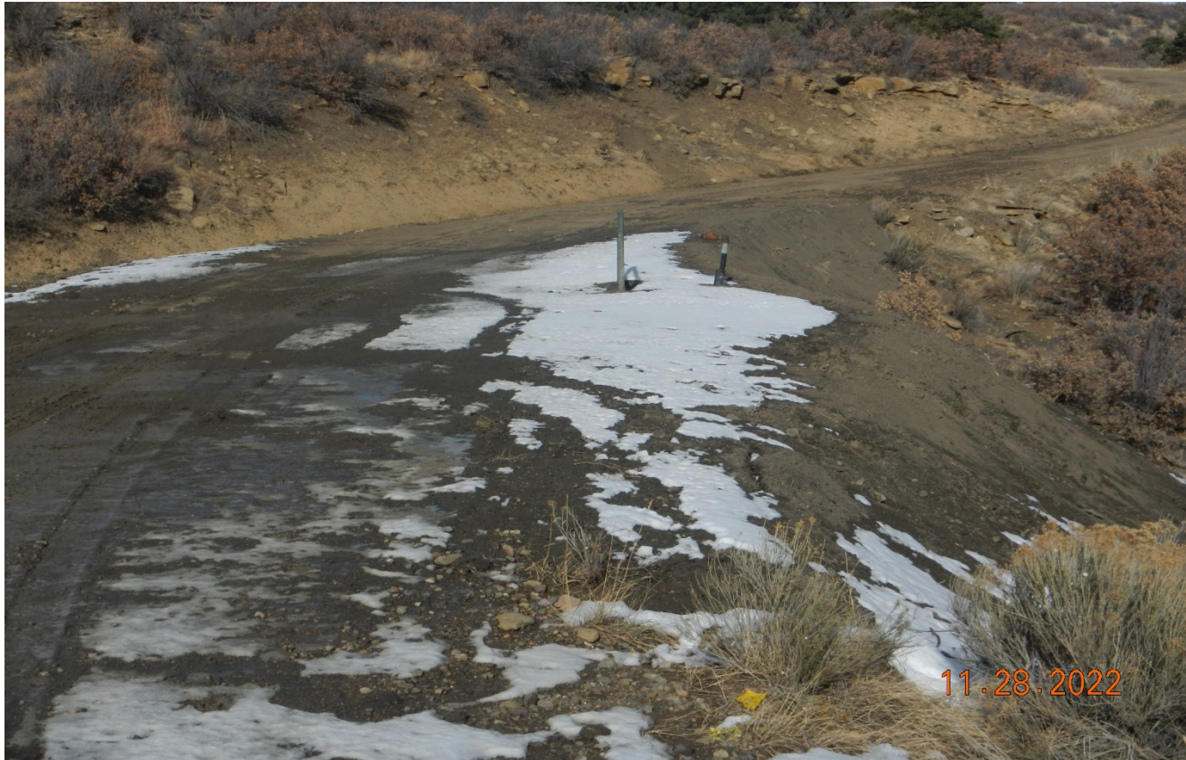
Photo 3. Facing back where the road was repaired. Loose soils along the embankment are susceptible to erosion.
