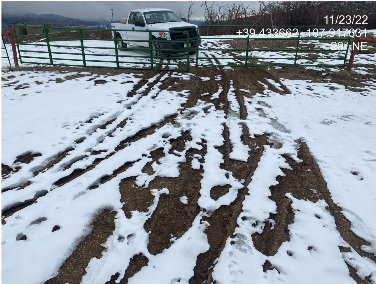
Photo 4. Photo shows degradation to pad surface at the entrance to the well production pad.
