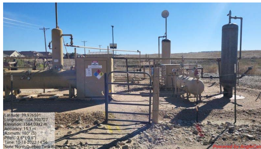
Photo 9 – Inadequate earthen secondary containment berm
