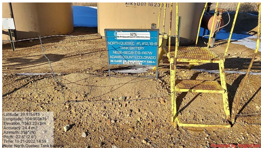
Photo 8 – Inadequate earthen secondary containment berm
