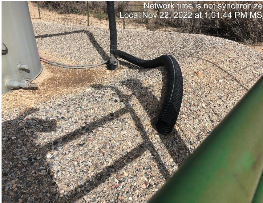
Photo #8506 Flowline heating insulation open ended.
