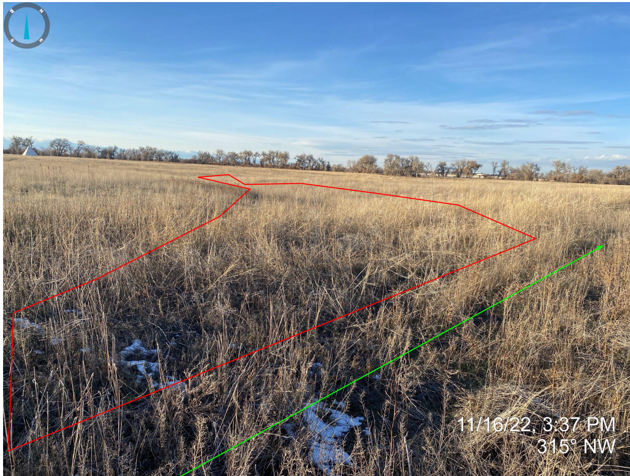
Photo 3. Taken from the access road, facing northwest. Photo illustrates the access road has not been recontoured to reflect reference areas. The portion of the access road appears to have been built in a natural swale and will need to be graded and contoured in order to meet final reclamation standards. Refer to Photo 5 for an aerial view. Green arrow shows approximate western edge of access road and direction of travel.
