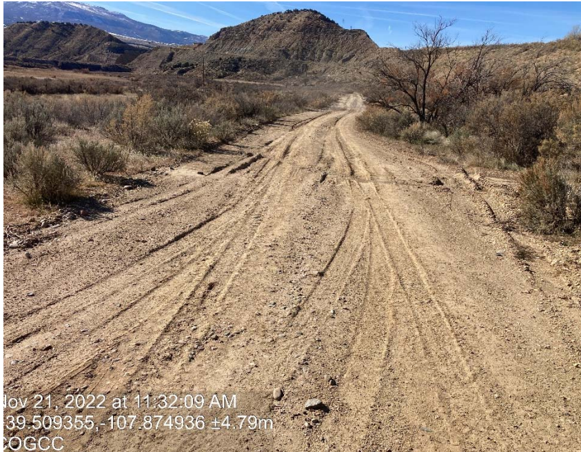
Access road erosion and lack of proper BMP's
