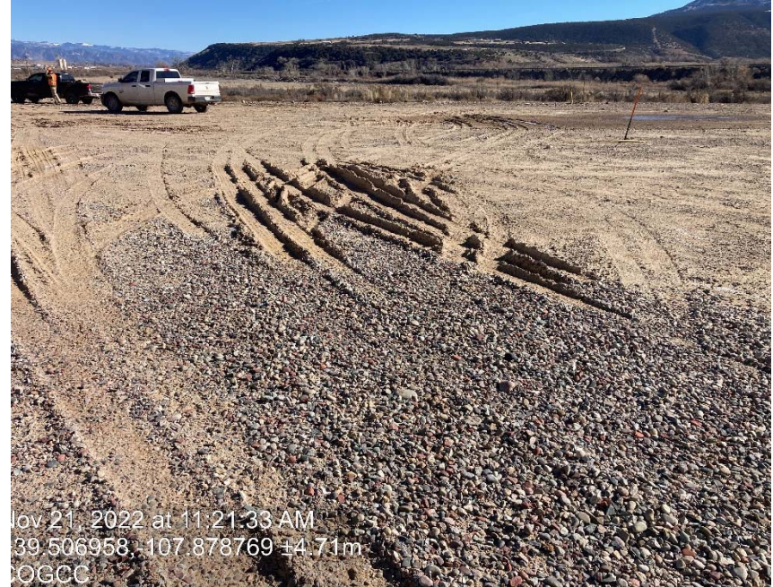
Lack of stabilization/ compaction
