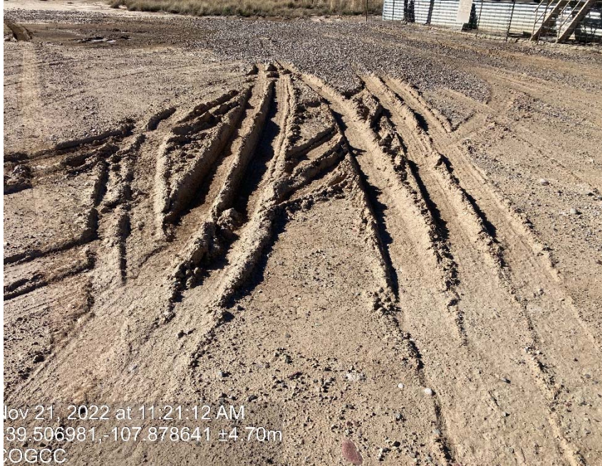
Lack of stabilization/ compaction
