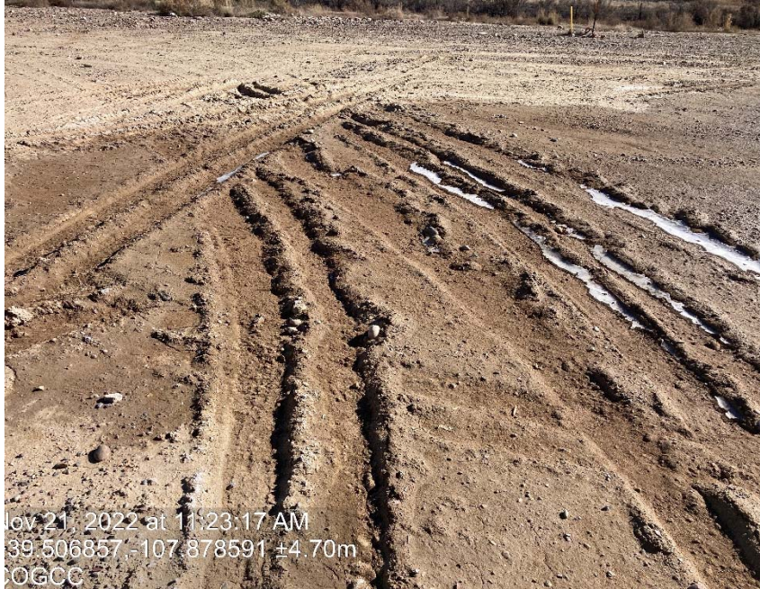
Lack of stabilization/ compaction
