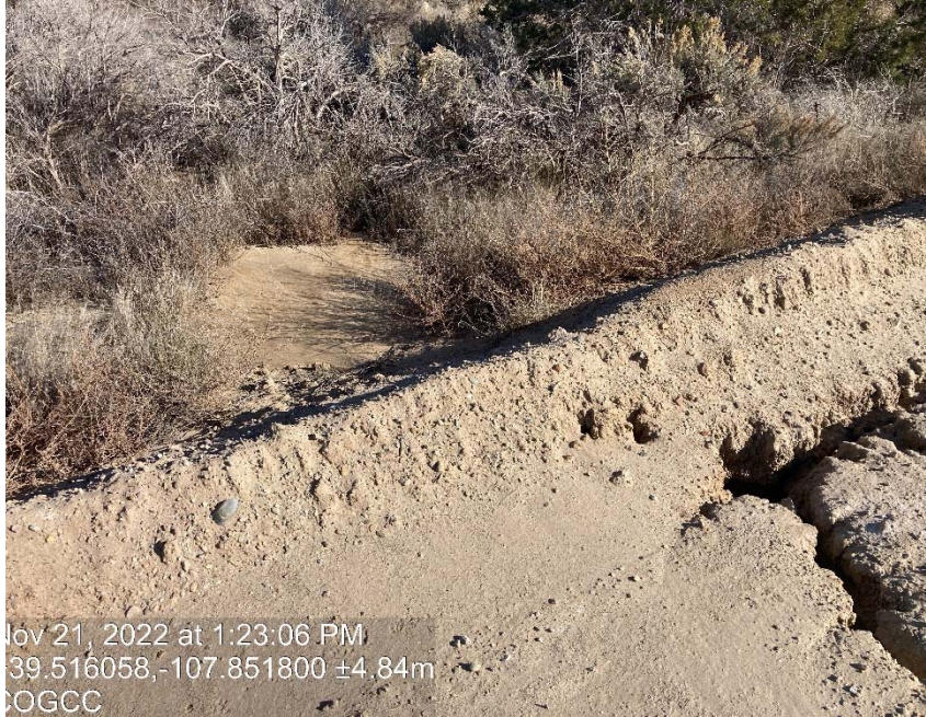
Erosion, tunneling through berm and sediment migration
