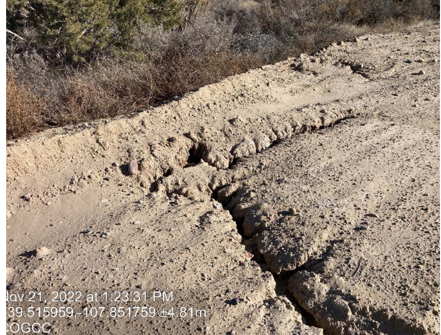
Erosion, tunneling through berm and sediment migration
