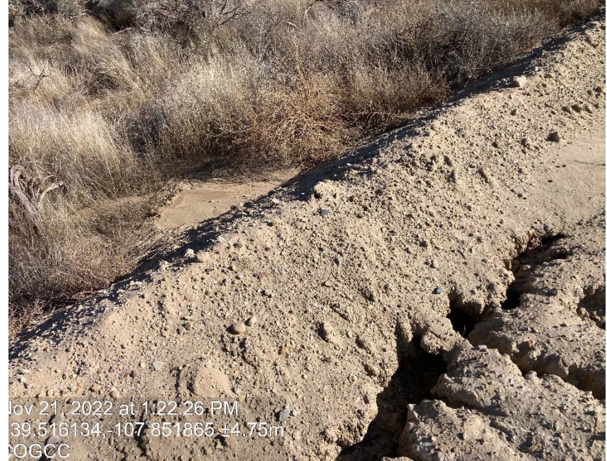
Erosion, tunneling through berm and sediment migration
