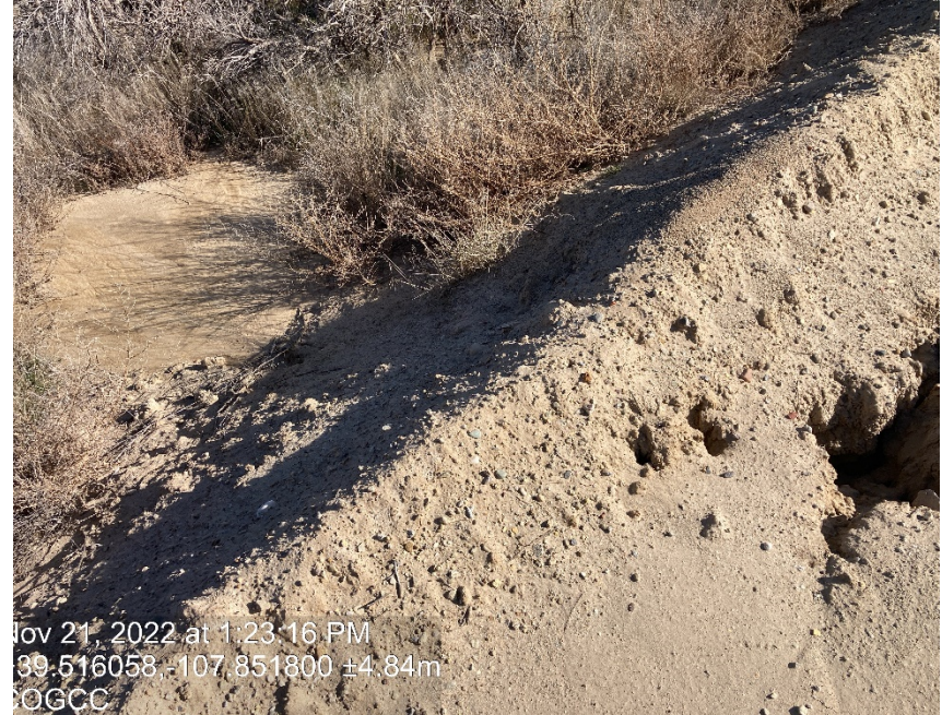
Erosion, tunneling through berm and sediment migration
