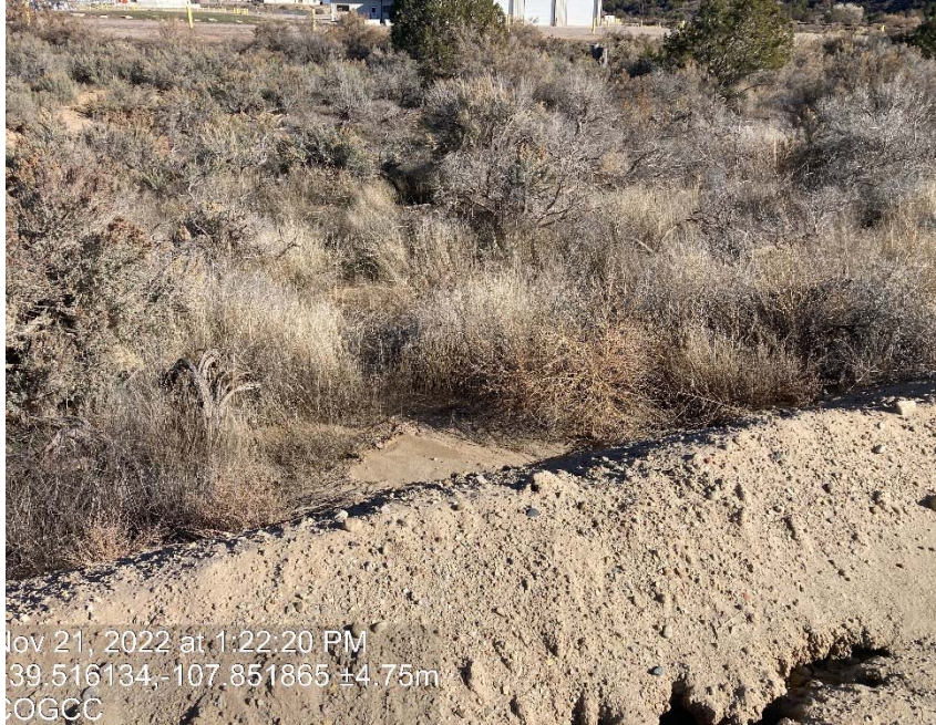
Erosion, tunneling through berm and sediment migration
