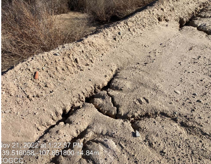
Erosion, tunneling through berm and sediment migration
