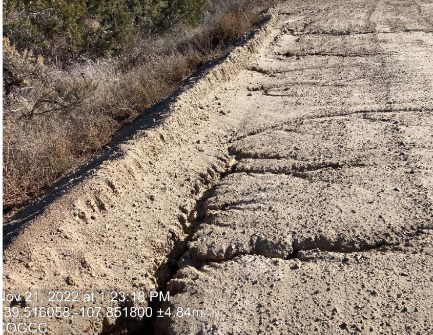
Erosion, tunneling through berm and sediment migration
