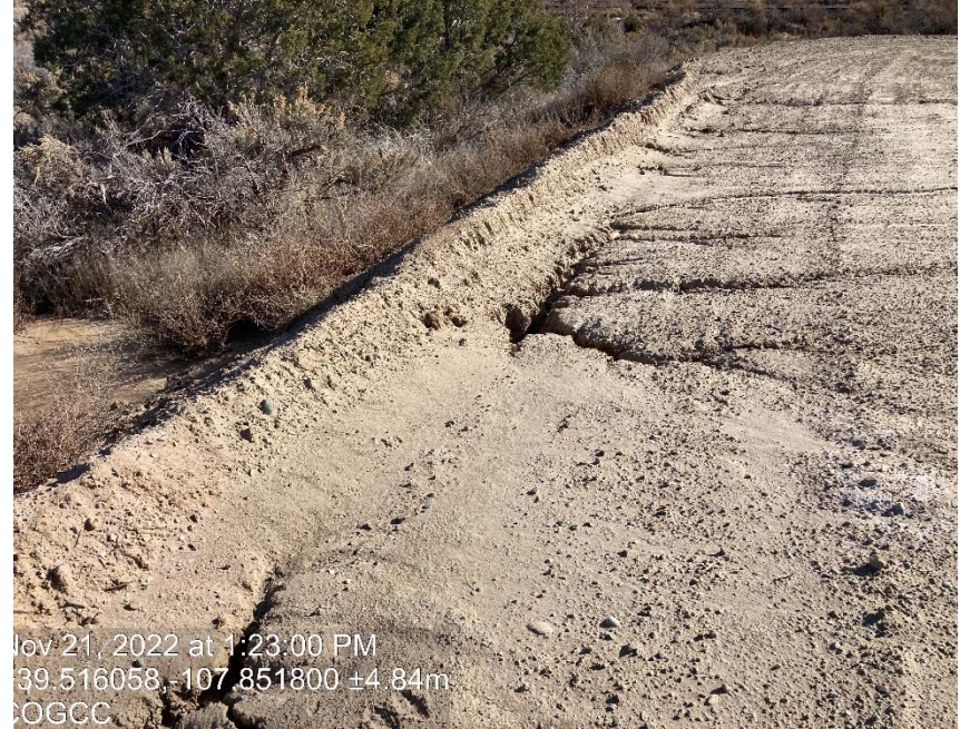
Erosion, tunneling through berm and sediment migration
