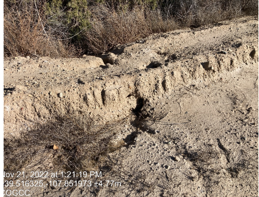
Erosion, tunneling through berm and sediment migration
