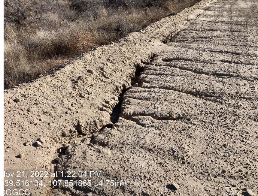
Erosion, tunneling through berm and sediment migration
