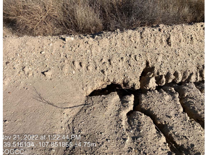
Erosion, tunneling through berm and sediment migration
