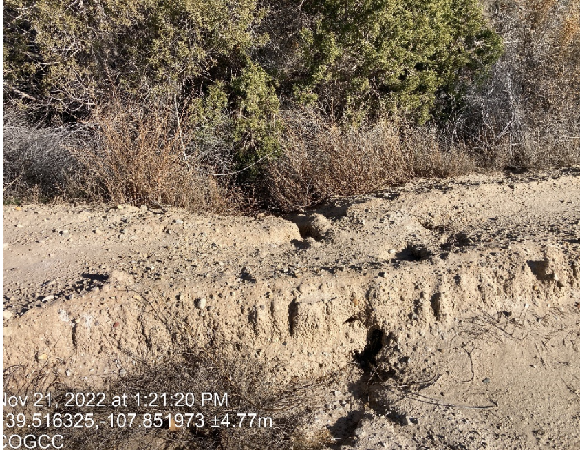
Erosion, tunneling through berm and sediment migration
