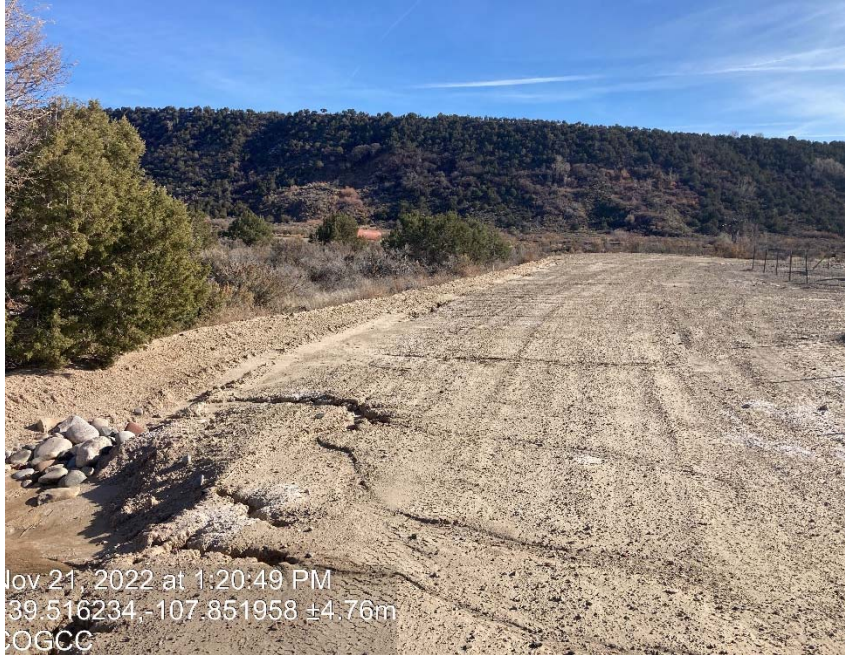
Erosion, tunneling through berm and sediment migration
