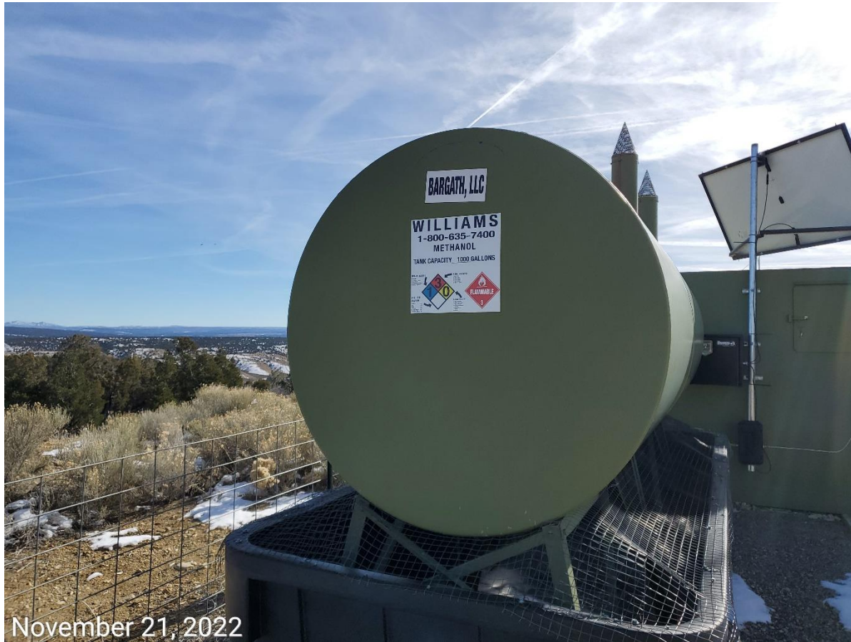
Photo 3: Photo of 1,000 gallon methanol tank. Photo shows Operator information is incorrect.
