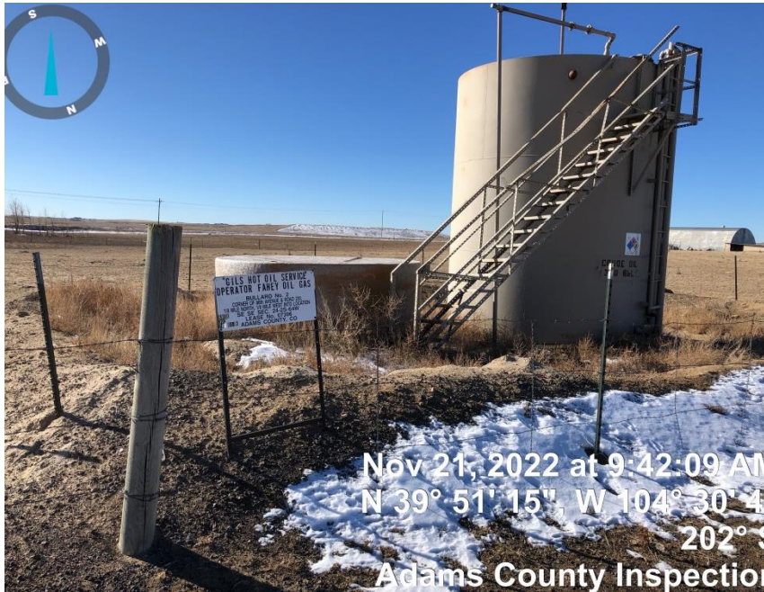
Photo#1 Production Tank and Produced Water Tank
