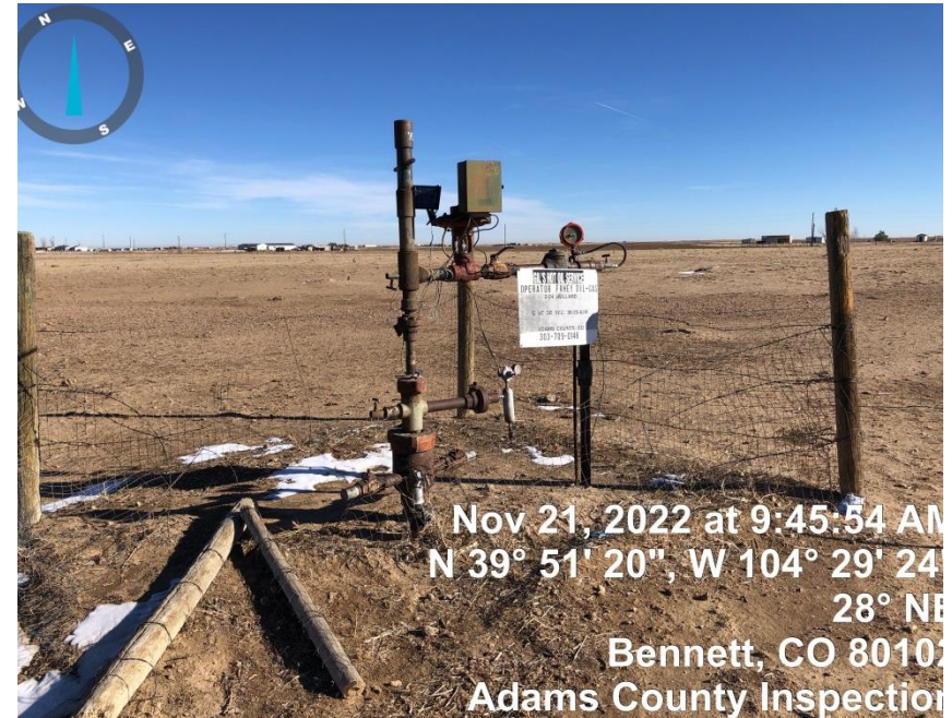
Photo#4 Wellhead Corrective Action/Fence In Disrepair
