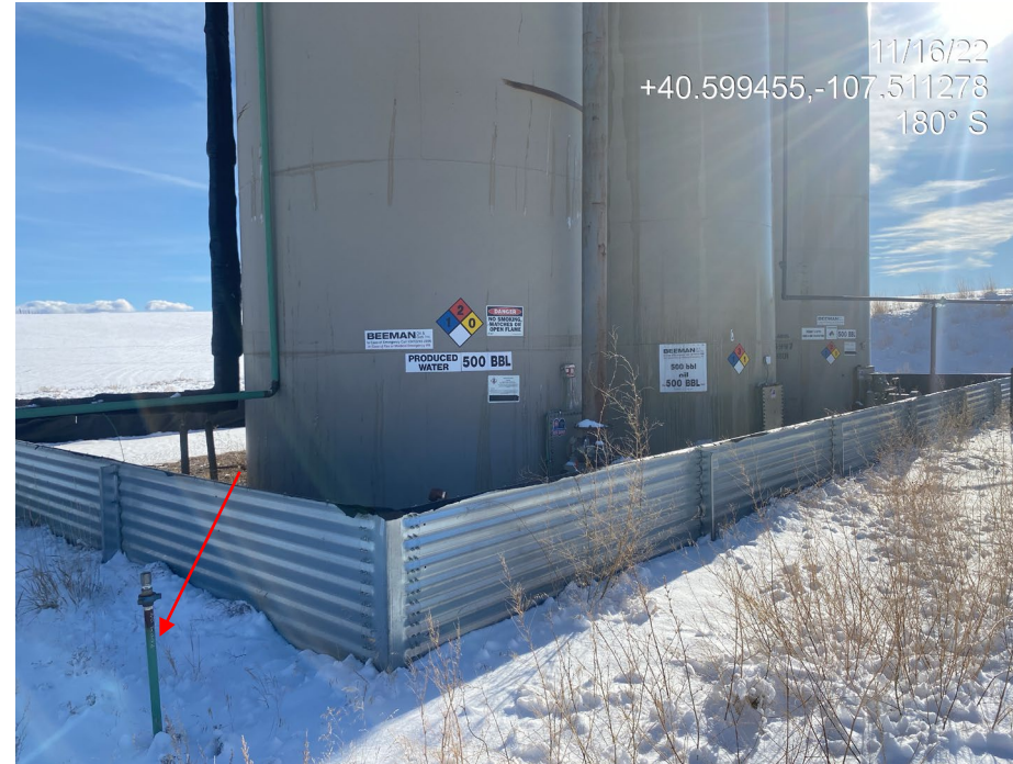
Photo 6. Photo shows an unused riser adjacent to the tank battery.
