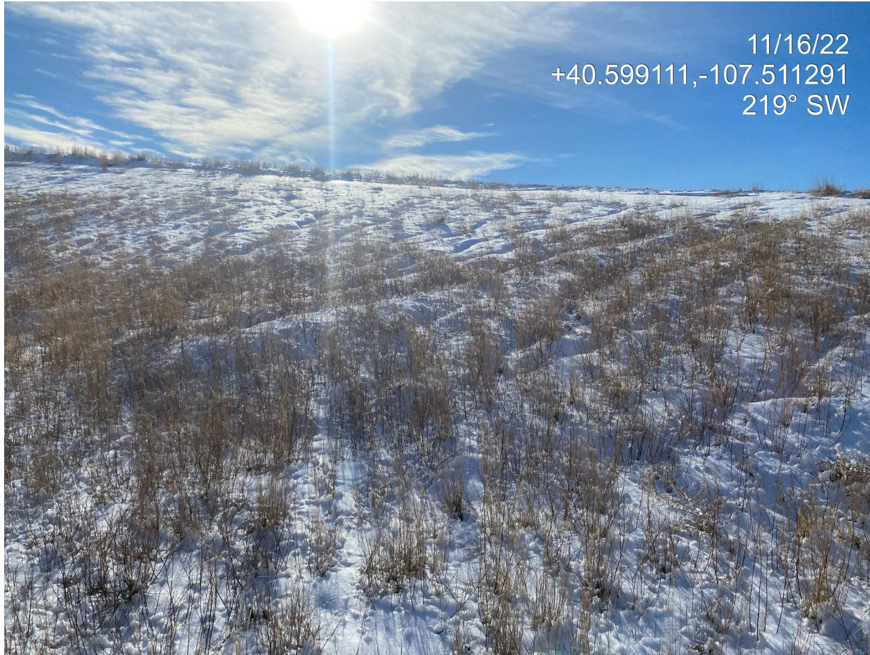
Photo 13. Photos taken from the cut slopes to the west of the Location shows widespread rill erosion occurring on slopes. Although snow cover obscures the slope, rills remain. There is no evidence the slope has been stabilized per previous corrective actions.
