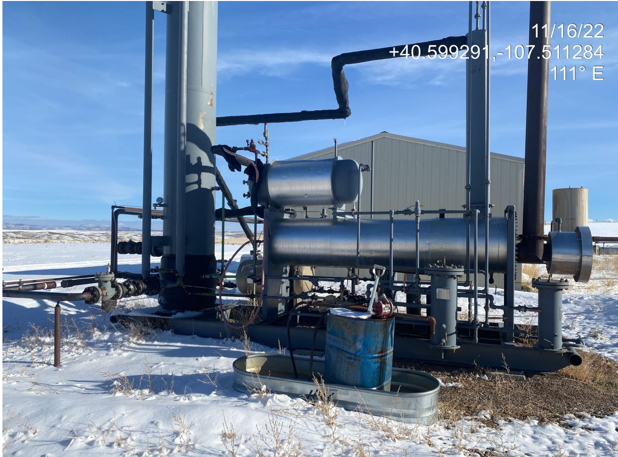
Photo 7. Photo taken from the west of the Location shows missing/insufficient wildlife protection BMPs on the secondary containment stock tank.
