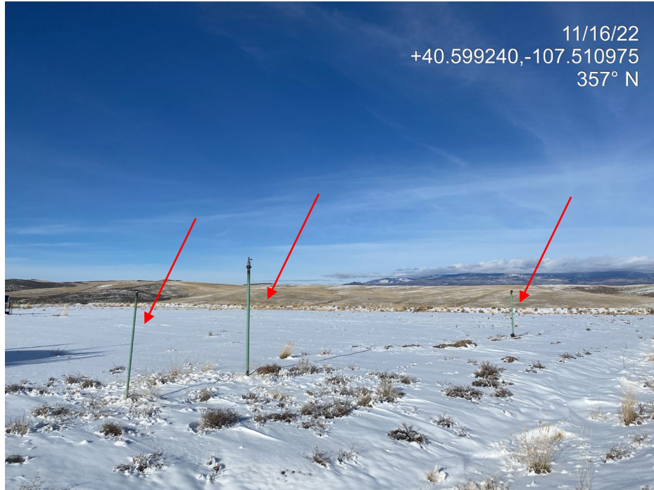
Photo 5. Photo shows unused risers at the south of the location.
