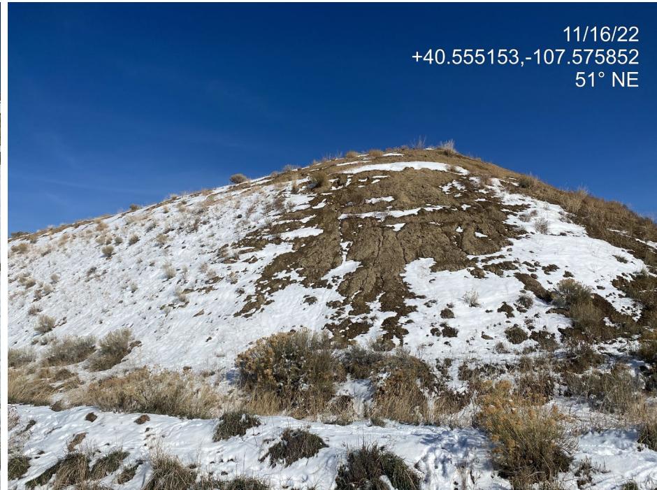
Photo 4. Photo taken from the southwest of the location shows cut slopes are bare and exposed. Rill erosion is evident.
