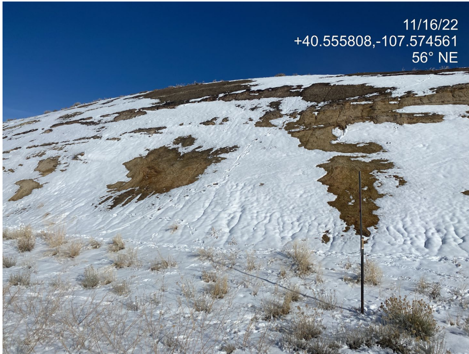
Photo 3. Photo taken from the east of the location shows cut slopes are bare and exposed. Rill erosion is evident.
