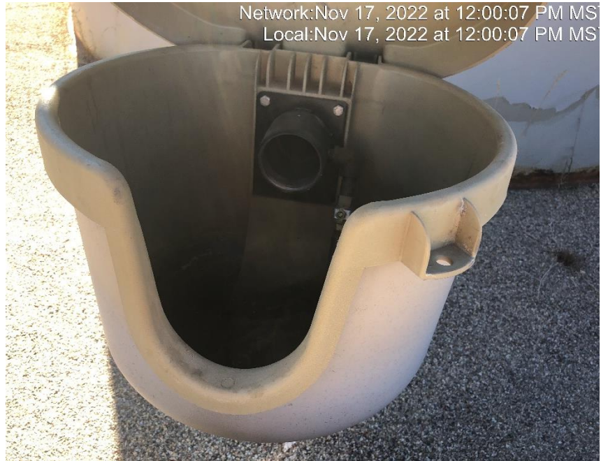
Photo #8431 Multiple loadlines open ended.
