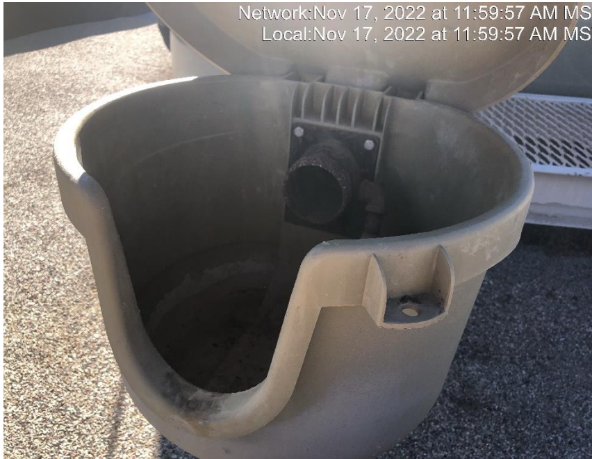
Photo #8429 Multiple loadlines open ended.
