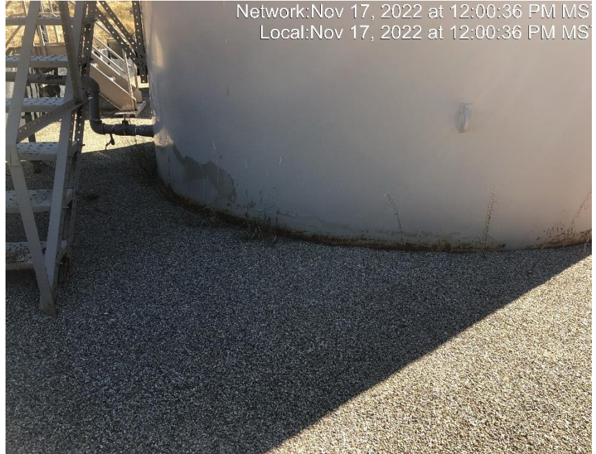
Photo #8433 Undesirable plant species in tank containment
