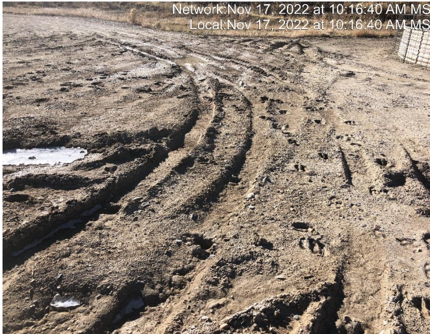
Photo #8405 Location lacks stabilization.
