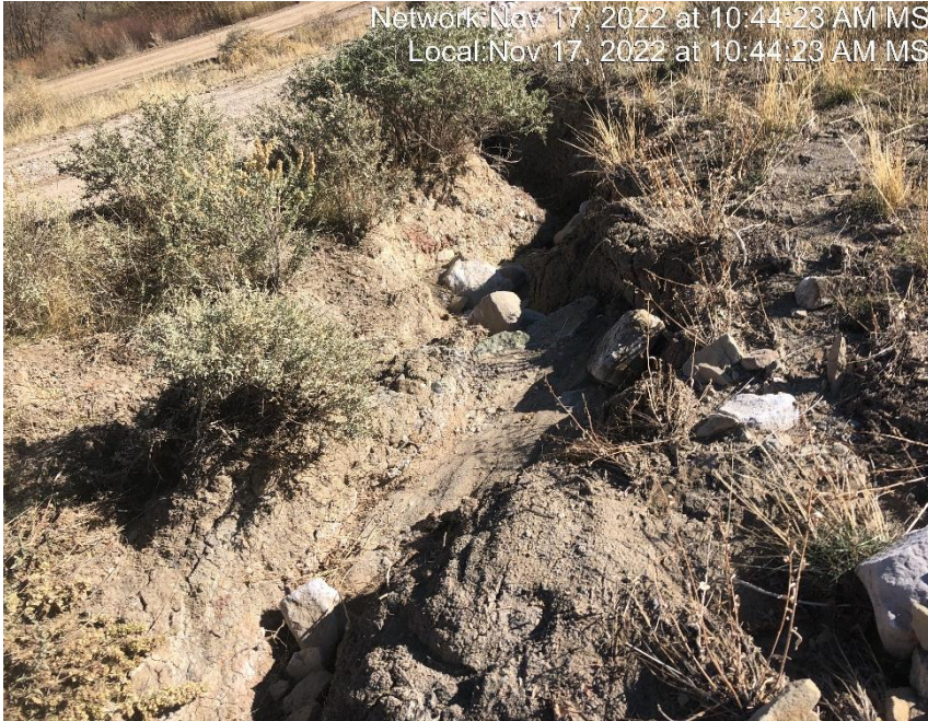
Photo #8414 Gully erosion occurring in access road ditch
