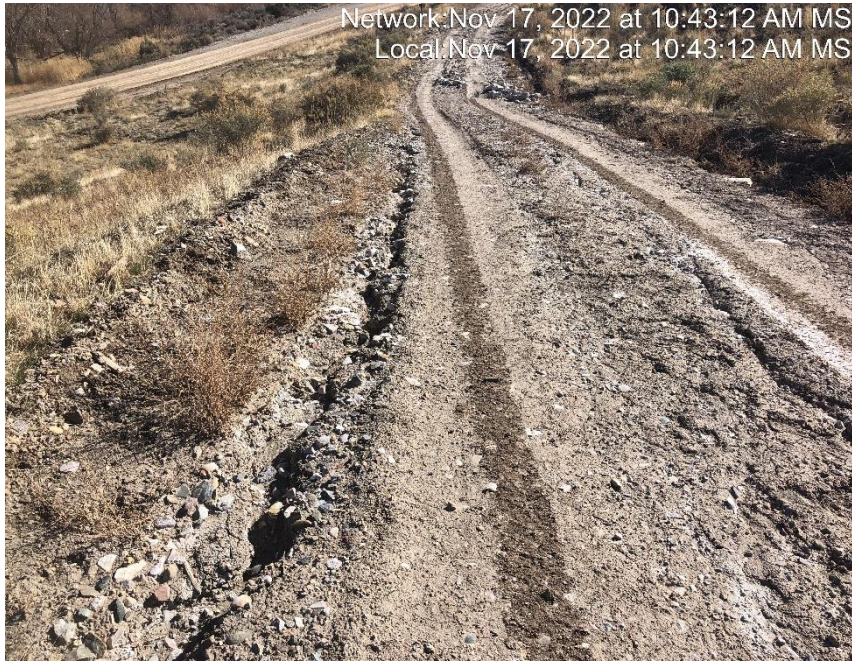
Photo #8409 Rill erosion occurring in access road.
