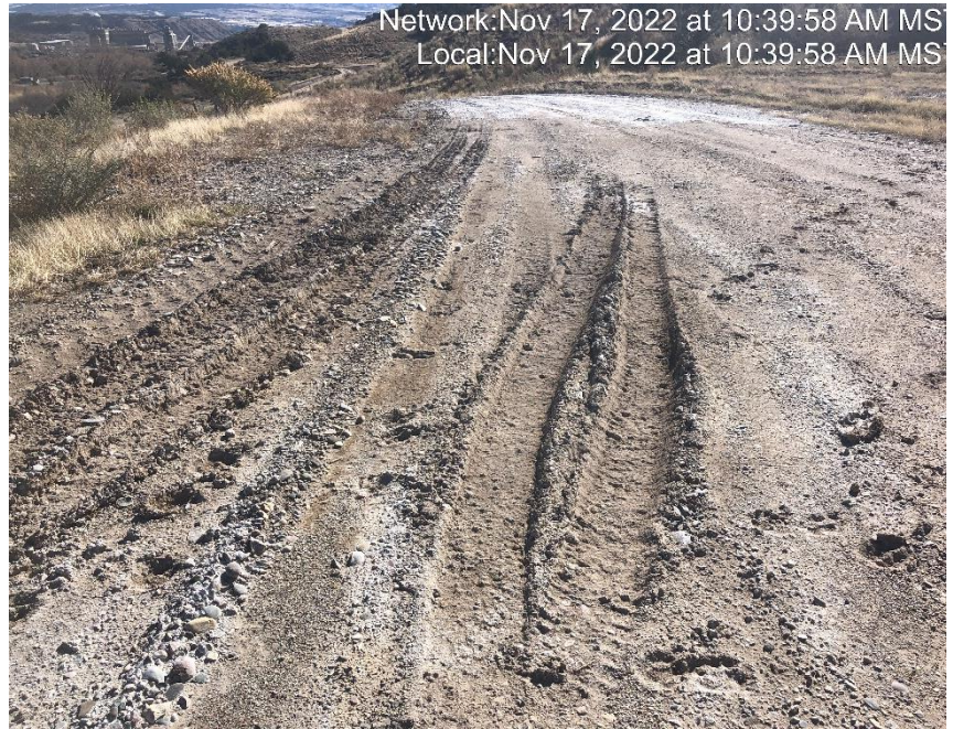
Photo #8407 Insufficient tracking BMP at entrance to location.
