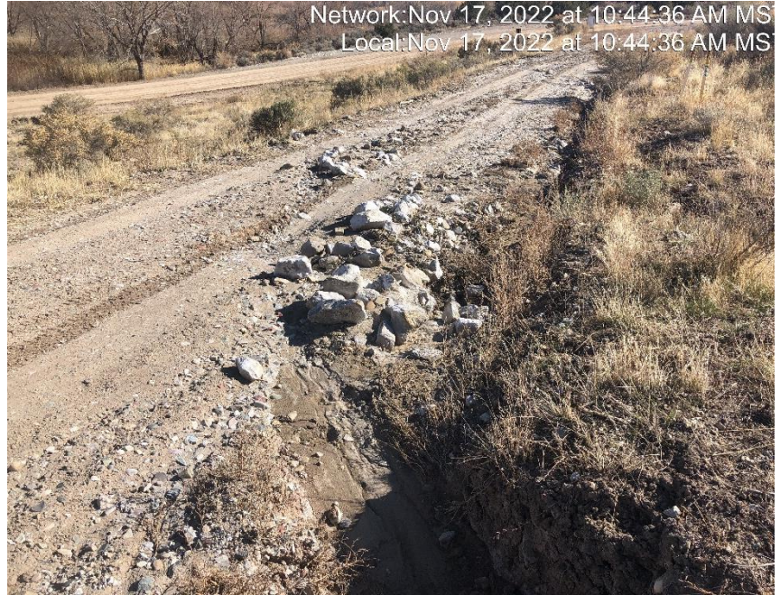
Photo #8415 Insufficient velocity checks.
