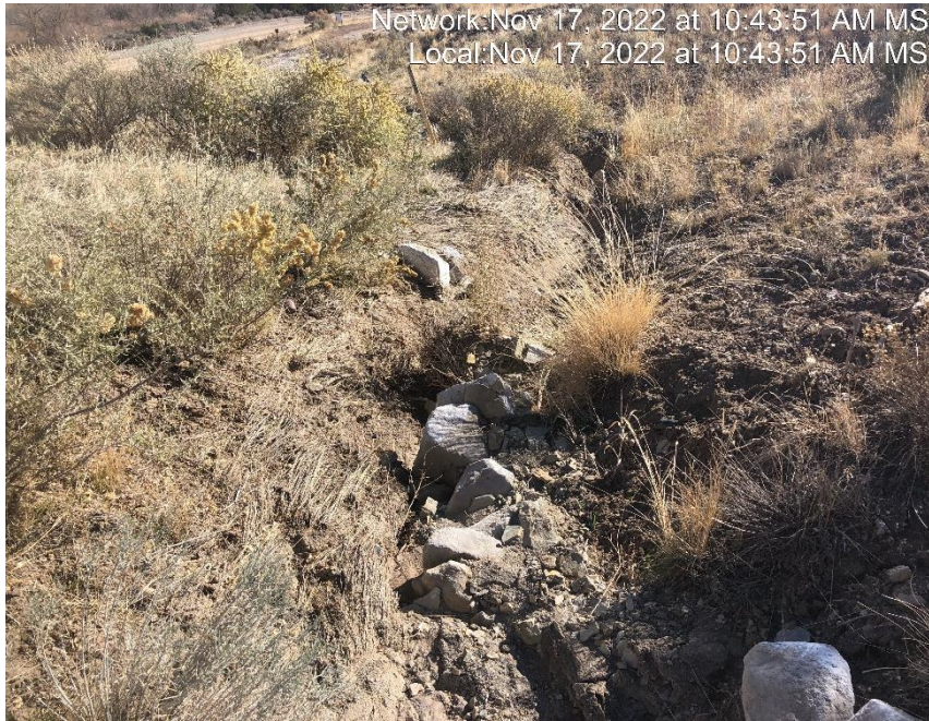
Photo #8411 Gully erosion occurring in access road ditch
