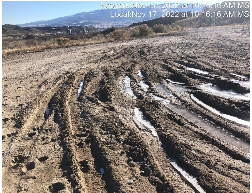
Photo #8404 Location lacks stabilization.
