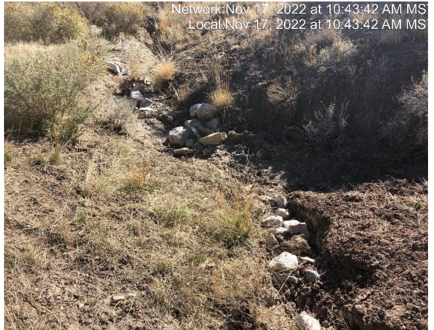
Photo #8410 Gully erosion occurring in access road ditch.
