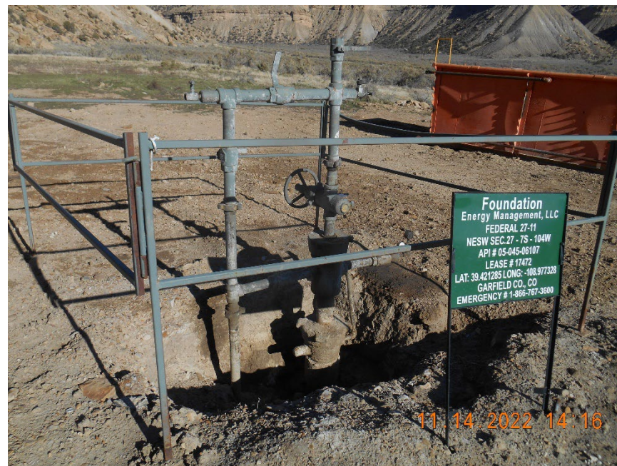
Wellhead with improper sign
