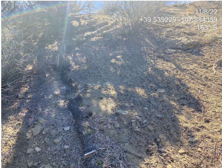
Photo 6. Photo shows an example of a perimeter wattle which is not in proper functioning condition; wattle is in disrepair (unstaked, losing straw) and sediment is overtopping the wattle.
