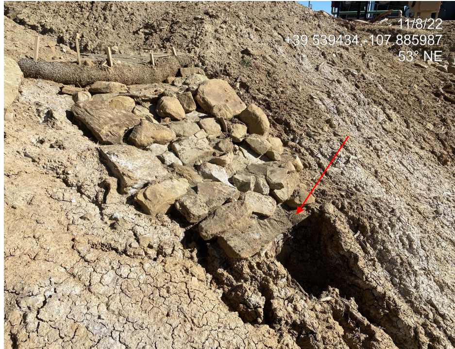
Photo 9. Photo shows a close-up of the ditch outlet/trap inlet in Photo 8. Degradation begins where a geotextile liner ends.
