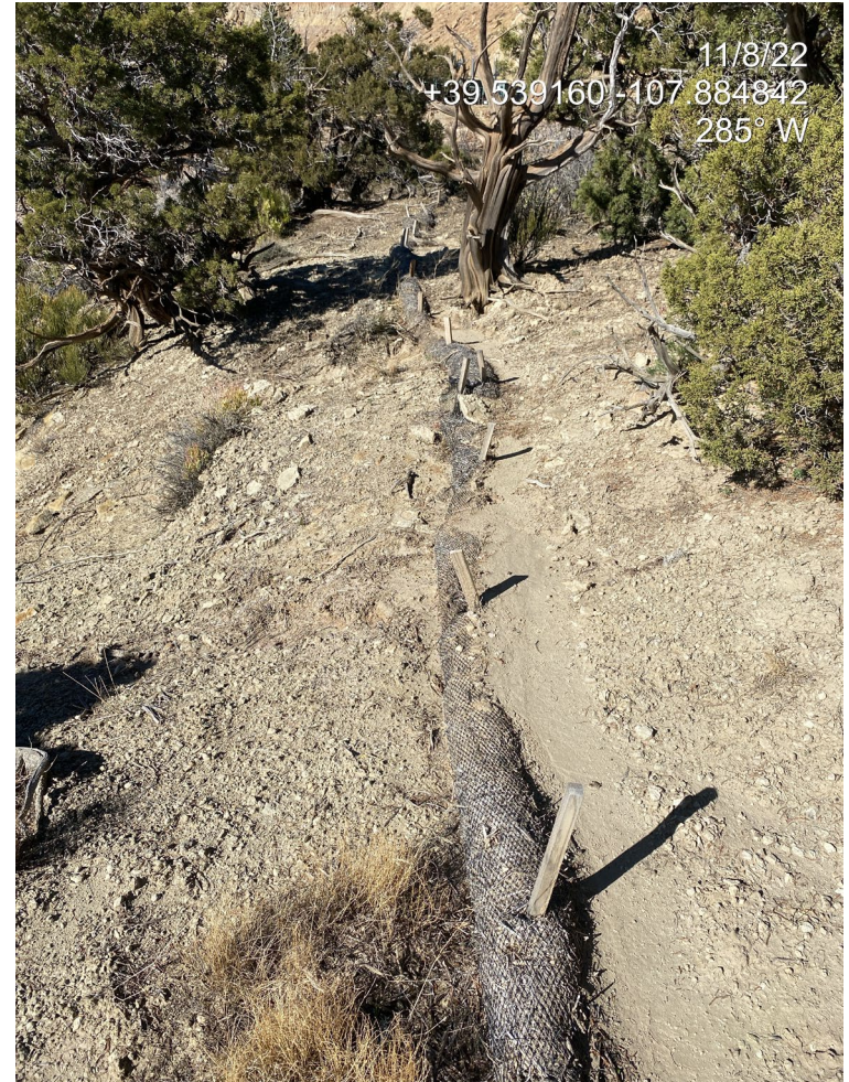
Photo 7. Photo shows an example of a wattle which is overwhelmed by sediment which is beginning to overtop the wattle.
