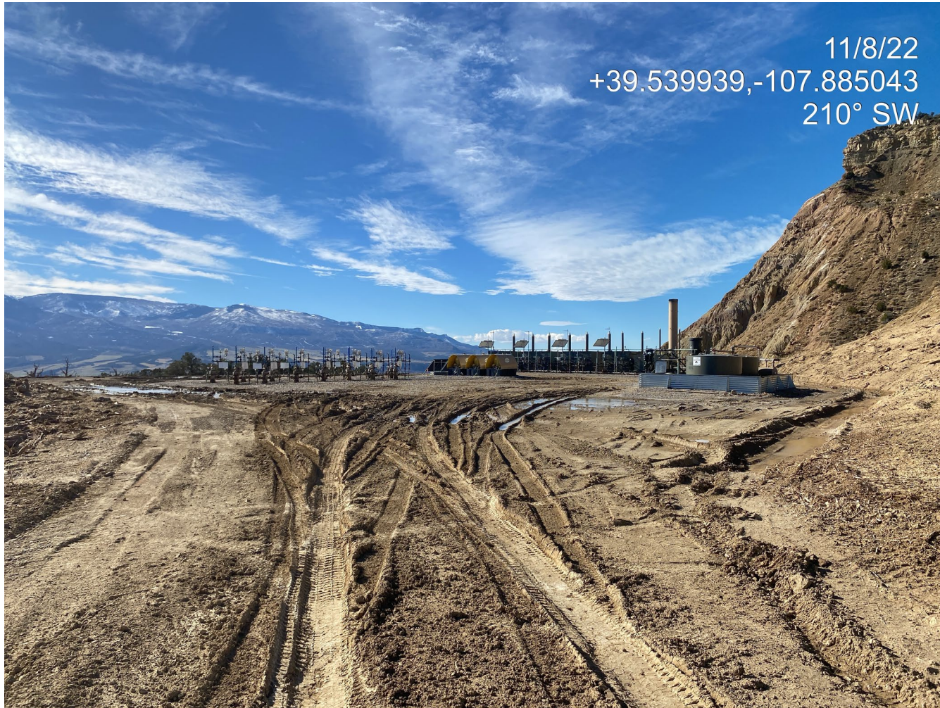
Photo 1. Photo taken from the location entrance shows an overview of the Location. Note pad surface compaction degradation.
