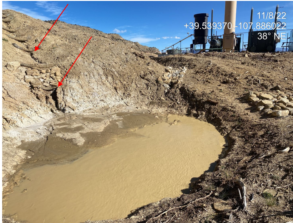
Photo 8. Photo shows where a diversion ditch enters a sediment trap at the west of the location. Degradation is occurring at the ditch outlet/trap inlet. Note also stormwater flows cutting beneath wattles in the diversion ditch. See Photos 10 and 11.
