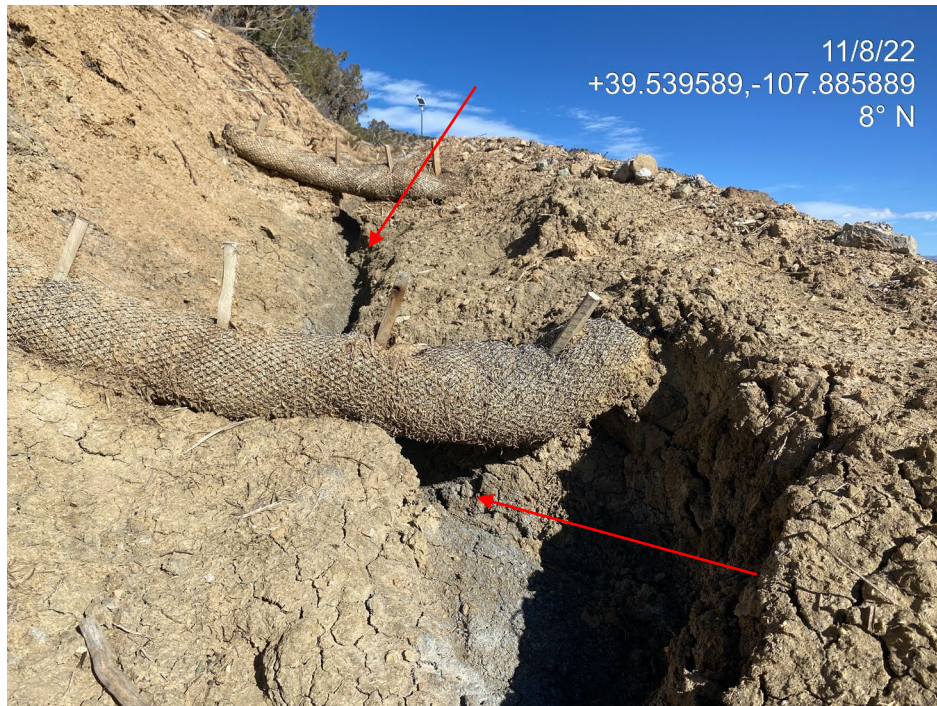
Photo 10. Photo shows degradation occurring in the diversion ditch at the northwest of the location. Concentrated flows are cutting beneath wattles in the ditch.
