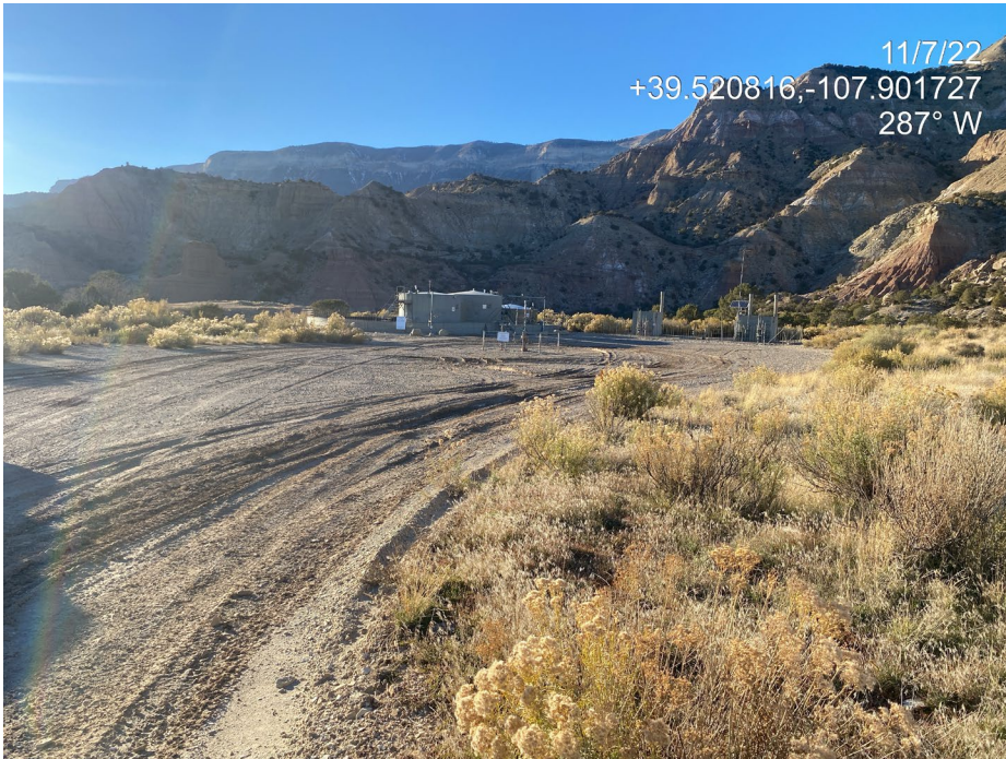
Photo 1. Photo shows an overview of the Location. Note pad showing lack of stabilization/compaction.
