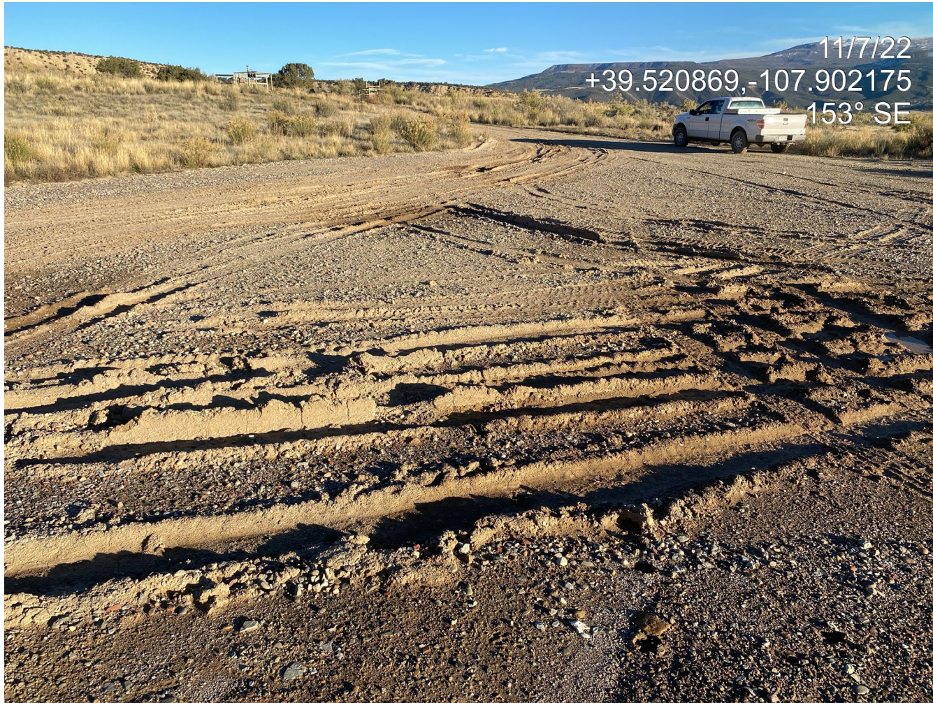
Photo 3. Note pad showing lack of pad stabilization/compaction.
