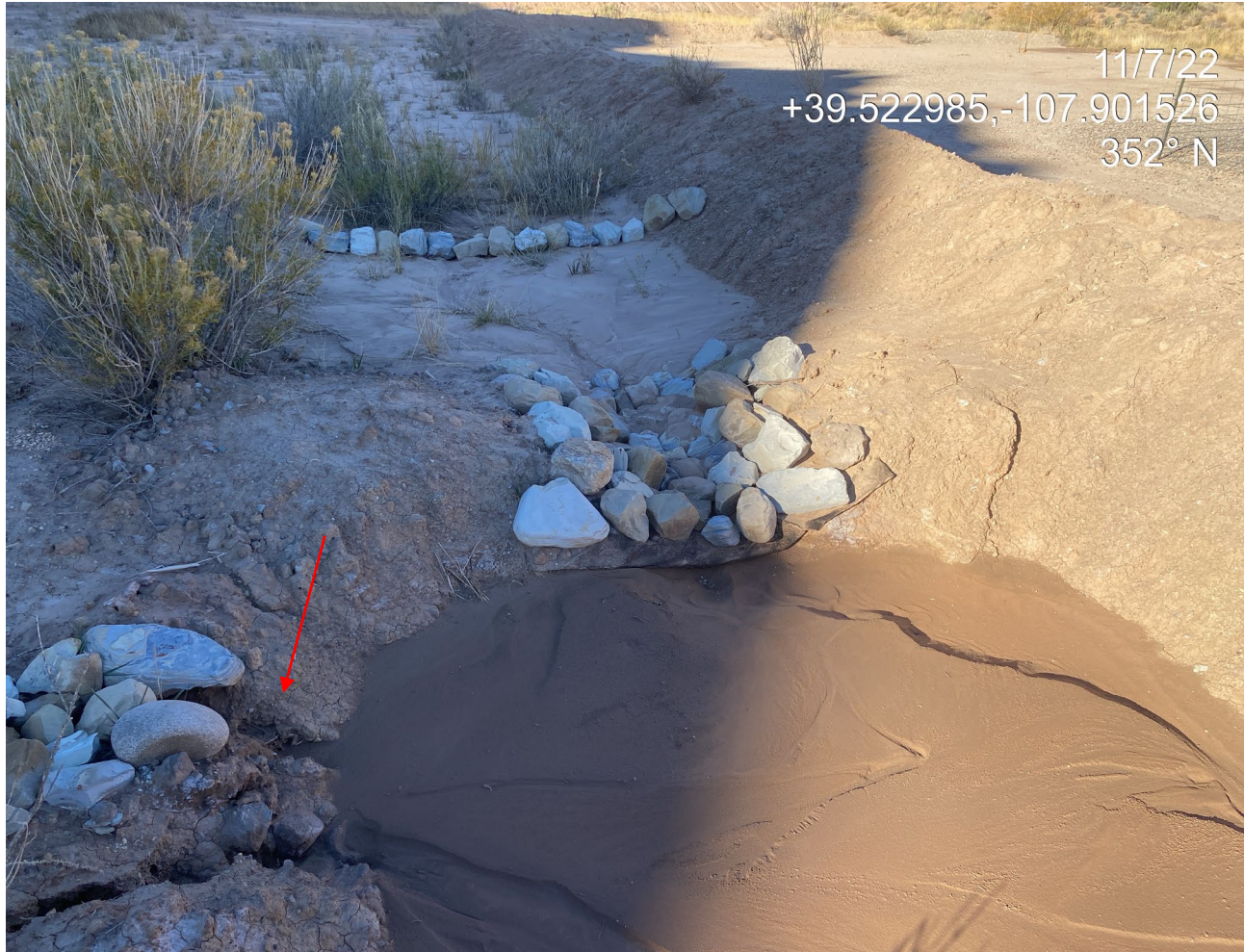
Photo 5. Photo shows stormwater BMPs at the west of the Location showing some signs of degradation; stormwater cutting beneath rocks, sediment traps approaching capacity.
