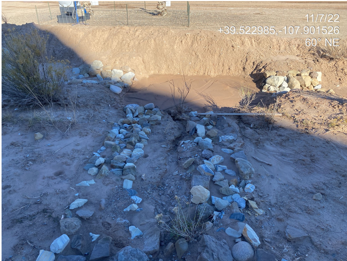
Photo 6. Photo shows stormwater BMPs at the west of the Location showing some signs of degradation; stormwater cutting through rocks, sediment traps approaching capacity.
