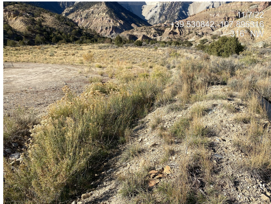
Photo 5. Photo shows taken from the east shows berms stabilized by perennial vegetation.
