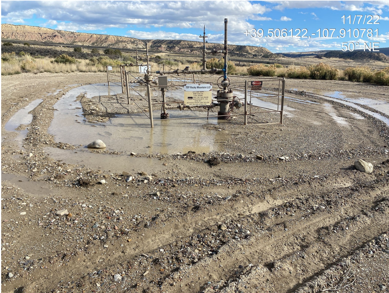
Photo 5. Photo shows lack of stabilization of the working pad surface.
