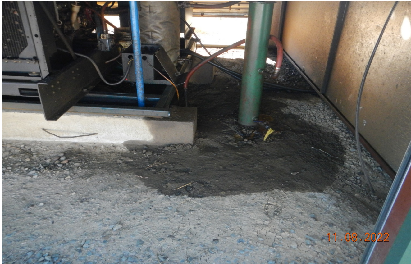
Photo 3. There is stained soils at the engine compressor that need to be cleaned up.
