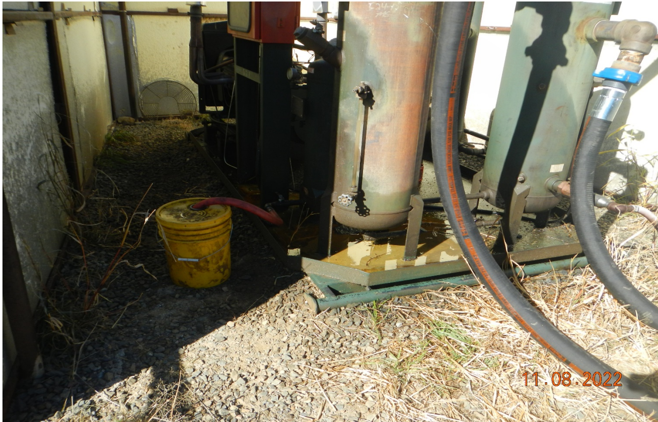
Photo 4. There is stained soils at the engine compressor that need to be cleaned up.
