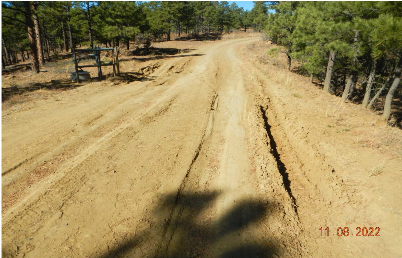
Photo 1. There is erosion and vehicle rutting along areas of the access road that will need to be repaired.
