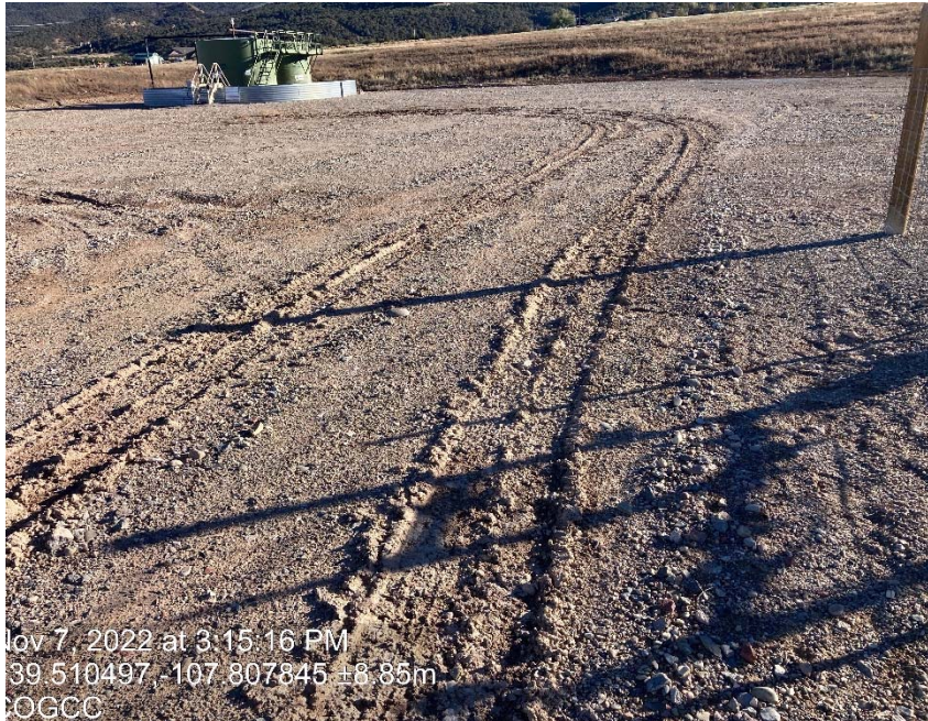
Lack of stabilization/compaction
