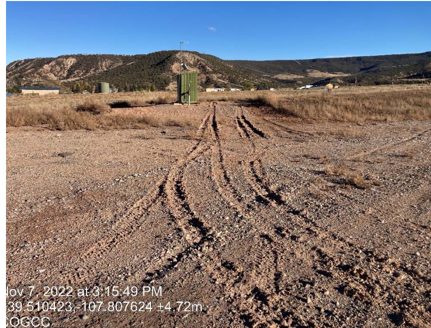
Lack of stabilization/compaction
