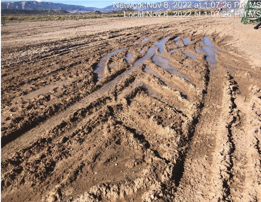
Photo #8345 Location lacks stabilization.
