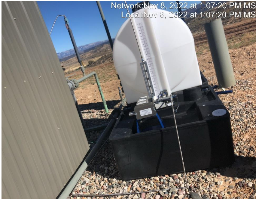
Photo #8344 Chemical tank missing required information.
