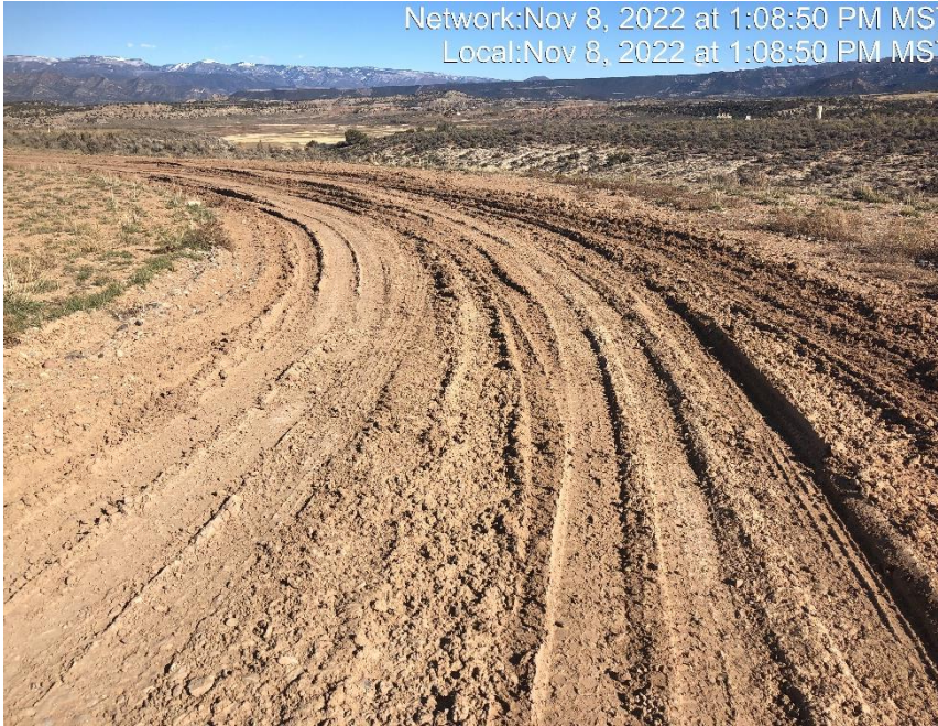
Photo #8349 Insufficnet tracking BMPs at entrance to location.
