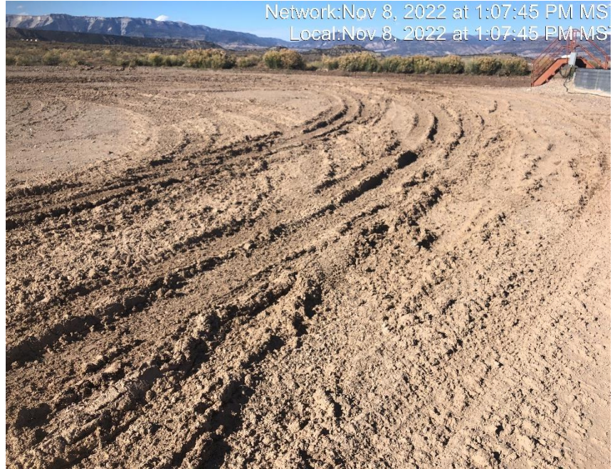
Photo #8346 Location lacks stabilization.
