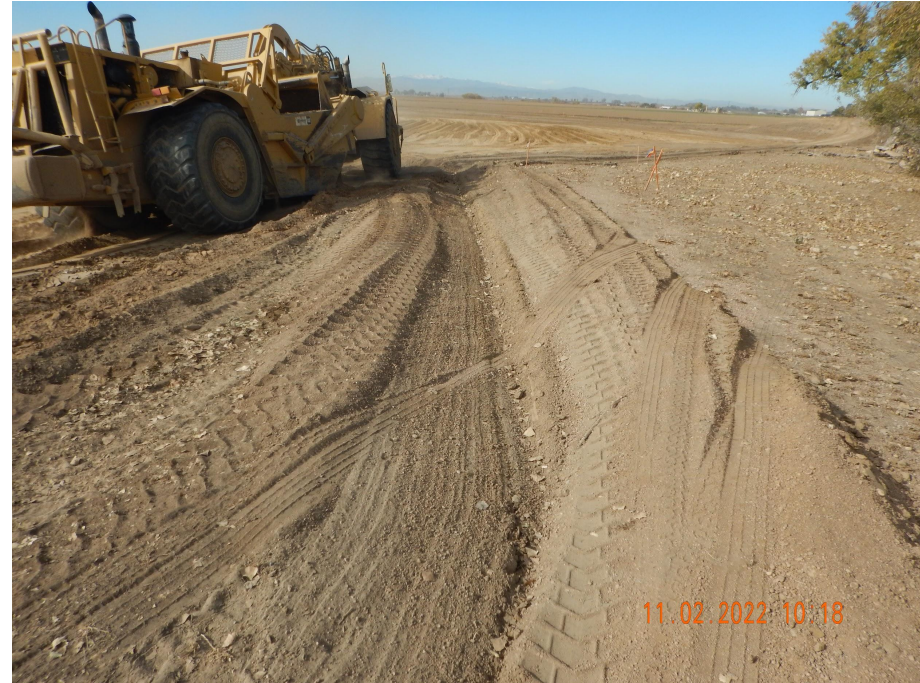
Photo 7. Photo taken from the northeastern location, facing West. Photo illustrates a ditch and berm BMP installed around the entire perimeter of location.
