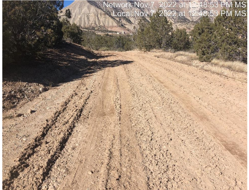
Photo #8318 Insufficient tracking BMP at entrance to location.
