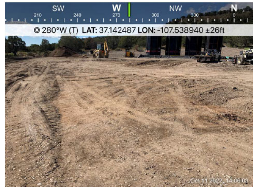
Photo 3: Area scraped and excavated following liner removal, 10/11/2022.
