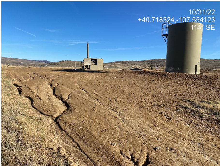
Photo 2. Photo taken from the Location entrance at the northwest shows erosion off the pad onto the access road.
