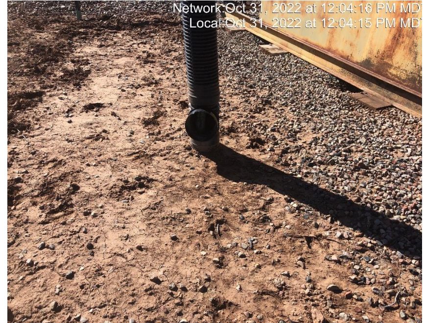
Photo #8260 Flowline heating insulation open ended and not capped.
