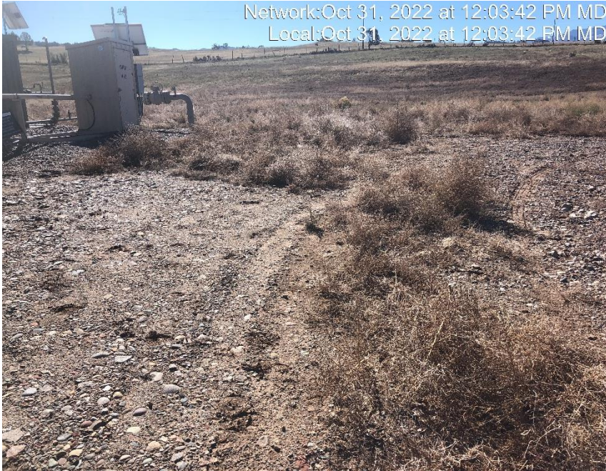
Photo #8259 Undesirable plant species in tank containment
